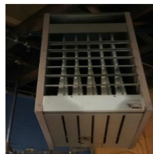
Hanging Gas-fired Furnace
