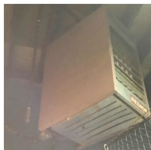
Hanging Gas-fired Furnace
