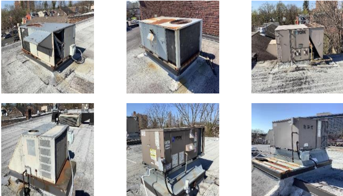
Roof Top Units (RTUs)
