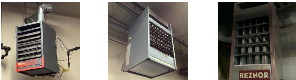
Gas-fired Unit Heaters
