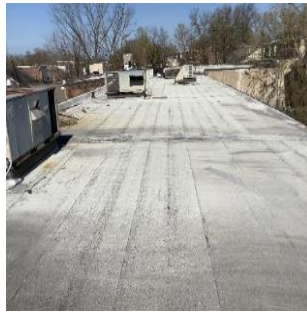
Flat Roof Section
