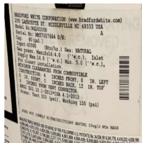
Gas-fired storage water heater
