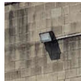
LED Wall Pack Fixtures
