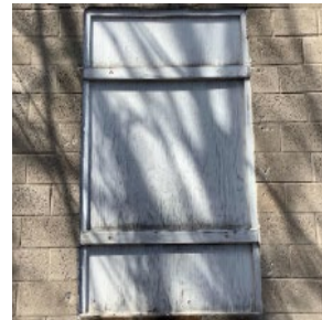
Boarded Window Opening
