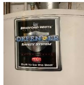
Gas-fired storage water heater
