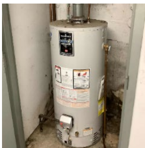
Gas-fired storage water heater
