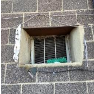
Exterior of AC Unit
