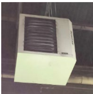
Suspended Gas-fired Furnace
