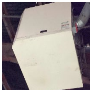
Suspended Gas-fired Furnace
