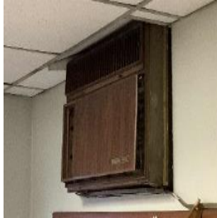
Interior of AC Unit in Office
