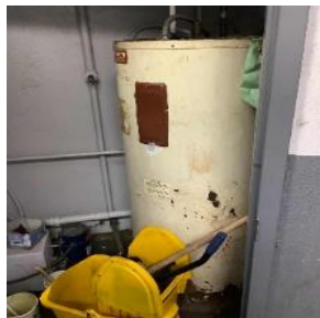
Domestic Hot Water Heater
