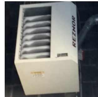
Suspended Gas-fired Furnace
