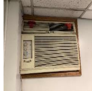
Interior of AC Unit in Office
