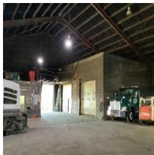
Interior Steel Truss
