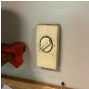
Electric Resistance Heater and Control
