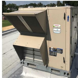
Typical Lennox Packaged Unit
