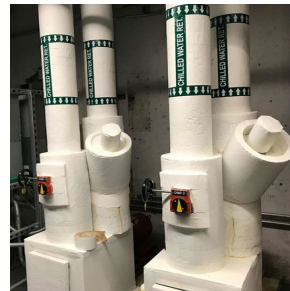
Chilled Water Pipes
