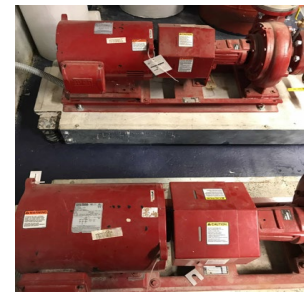
15 hp Variable Flow Hot Water Pumps
