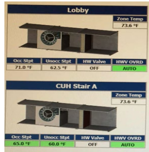
BEMS Screenshot - Hydronic Unit Heaters
