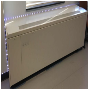
Typical Classroom Unit Ventilator
