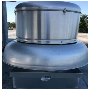
Typical General Exhaust Fan
