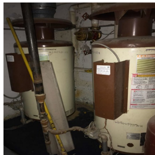
Domestic Hot Water Boilers
