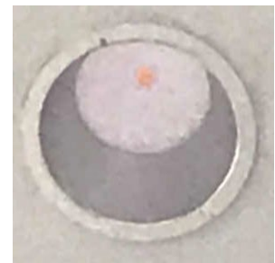
Exterior LED Fixtures
