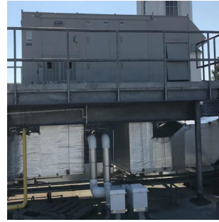
AHU-1/Chilled Water and Gas Pipes
