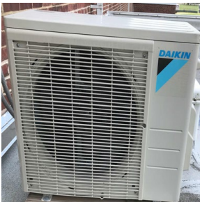
Outdoor Daikin Split System AC
