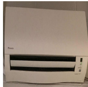
Indoor Daikin Split System AC
