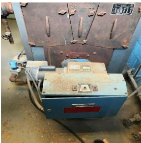
Non-condensing Hot Water Boiler
