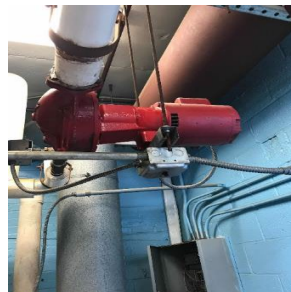
Heating Hot Water Pump
