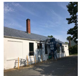
Façade and Roof
