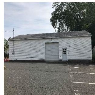
Building Façade and Roof
