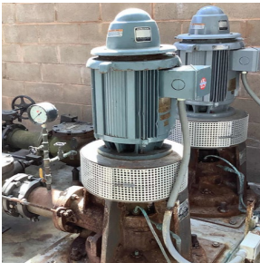
Water Wash Pumps
