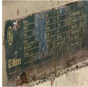
Thickener Sludge Pumps
