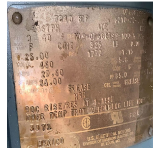
Water Wash Pumps
