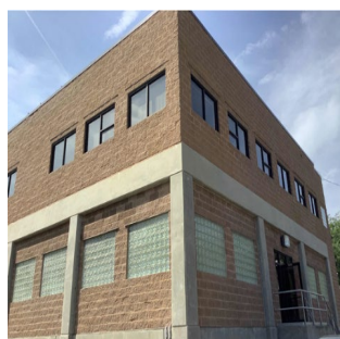
Main Office Building
