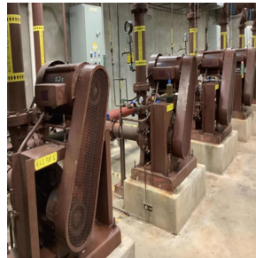
Return and Waste Sludge Pumps
