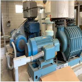
150 hp Aeration Blowers (Positive Displacement Blower #2)
