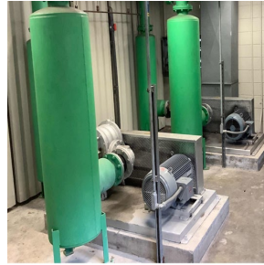
Anaerobic Sludge Storage Blowers
