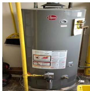
Storage Tank Water Heater
