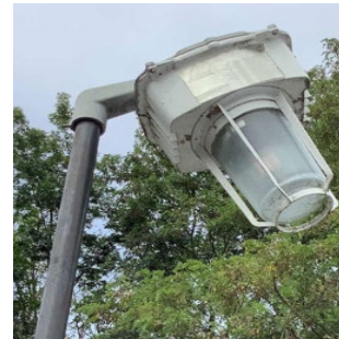
Pole Mounted Fixture
