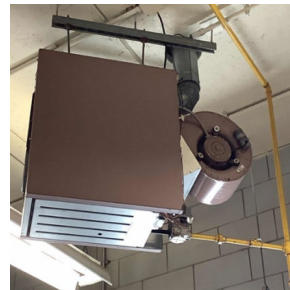
Typical Reznor Unit Heater
