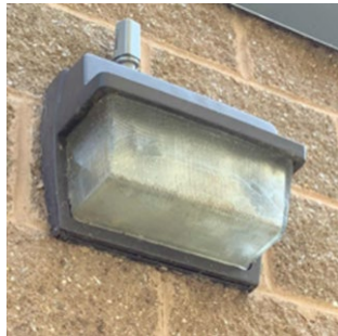
Exterior Wall Fixture
