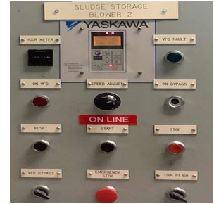
Anaerobic Sludge Storage Blowers
