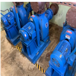
Raw Sewage Pumps
