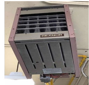
Typical Reznor Unit Heater
