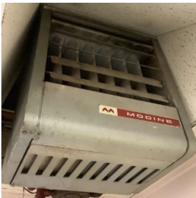
Garage Bay Modine Unit Heater
