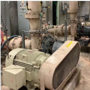
Internal Recycling Pumps
