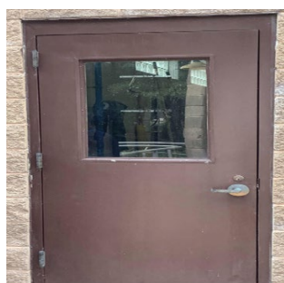
Alum Building Exterior Door
