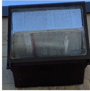
HID Wall Mounted Fixture
