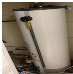
Storage Tank Water Heater
