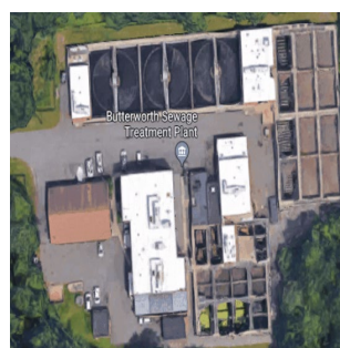
Butterworth Sewer Treatment Plant Aerial View
