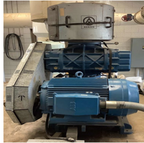
150 hp Aeration Blowers (Positive Displacement Blower #2)
