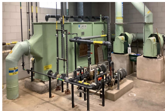
Scrubber Recirculation Pumps & Exhaust Air Fans
