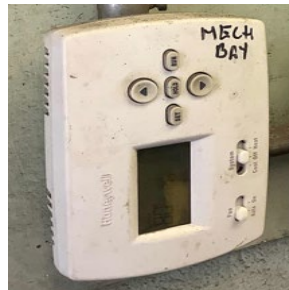
Garage Bay Modine Unit Heater Control
