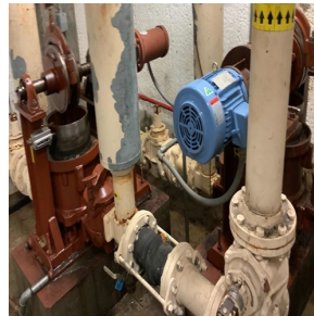
SCUM Storage Pump
