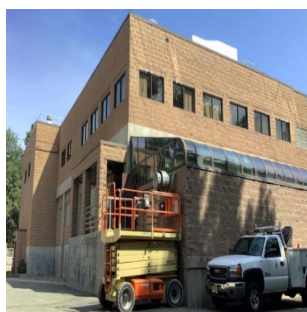
Main Office Building
