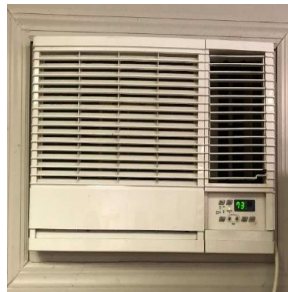
Window AC Unit
