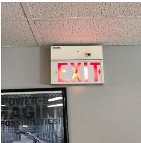
Non-LED Exit Sign
