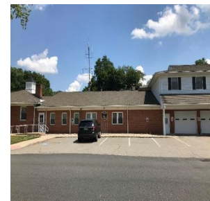
Left-Side of the Building
