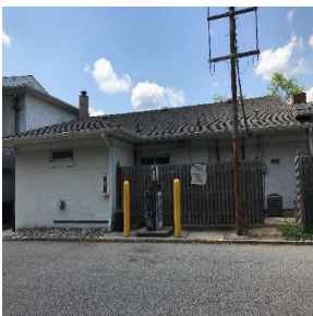
Right-Side of the Building
