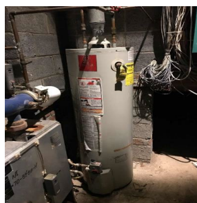
Gas-Fired Storage Water Heater
