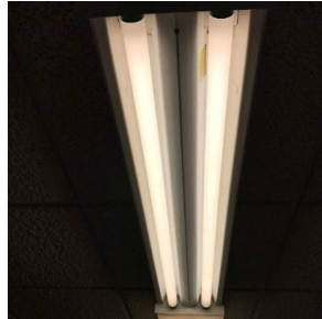
Fluorescent T12 Fixture
