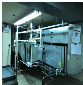
One of the AHU's
