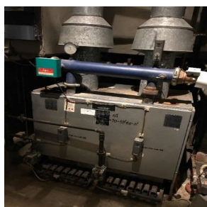
First-Floor Hot Water Boiler
