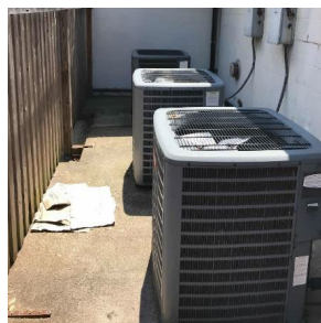
Outdoor Condensing Units
