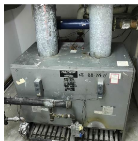
Second-Floor Hot Water Boiler
