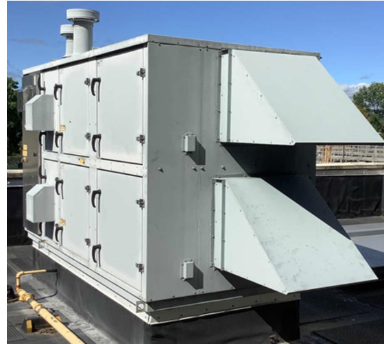
New Reznor & Two Stage Heatco Heating Furnace
