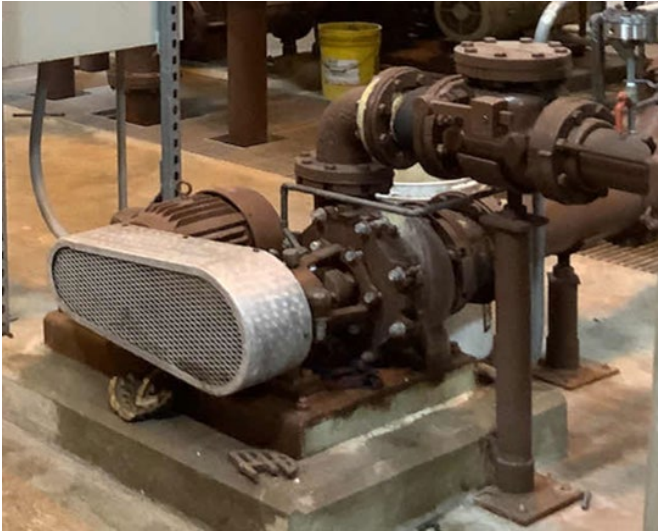
Waste Activated Sludge Pump #3
