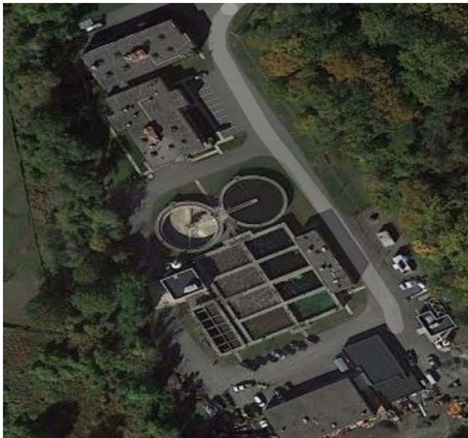
Woodland Sewer Treatment Plant Aerial View
