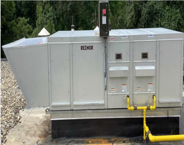
New Reznor & Two Stage Heatco Heating Furnace
