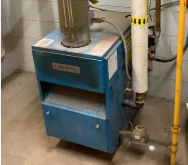
Non-Condensing Hot Water Boiler & 0.8 hp Hot Water Pumps
