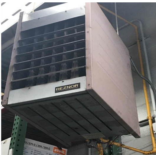
Gas-Fired Unit Heater & Local Thermostat
