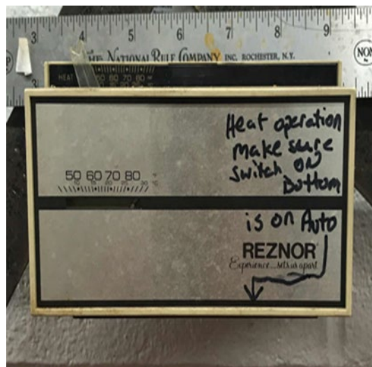
Gas-Fired Unit Heater & Local Thermostat
