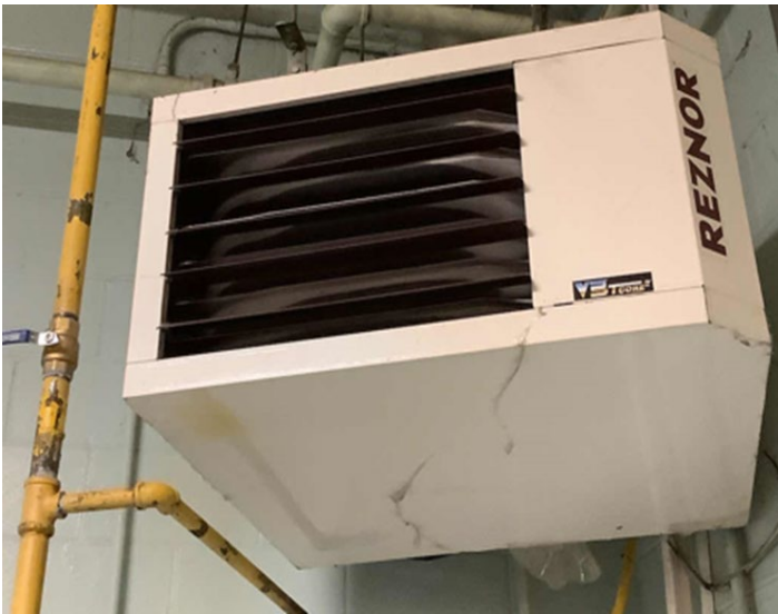
Gas-Fired & Electric Resistance Heaters
