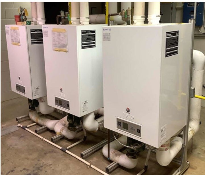
Condensing Hot Water Boilers
