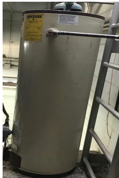
50 & 40 Gallon Storage Tank Water Heaters
