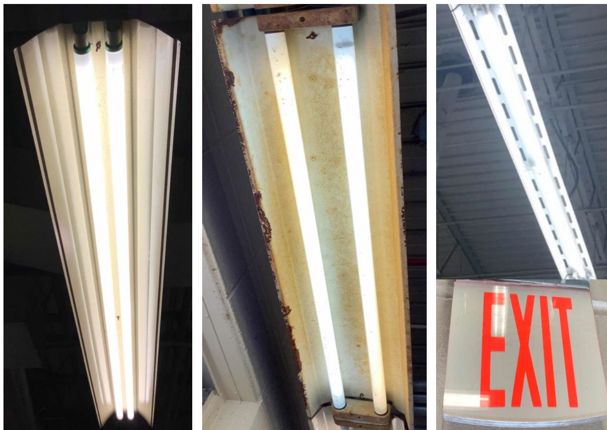
8-Foot Linear T12, 4-Foot T5, & LED Exit Sign
