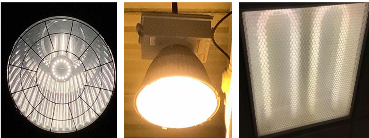
LED Corn Bulb, HID, & U-Bend T12 Fixture
