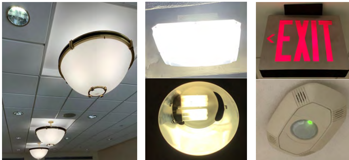
CFL, LED, LED Exit Sign & Wall Mounted Occupancy Sensor
