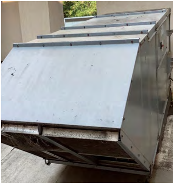
MUA-1 & Electric Resistance Heater
