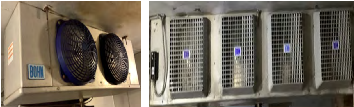
Walk-in Indoor Evaporators
