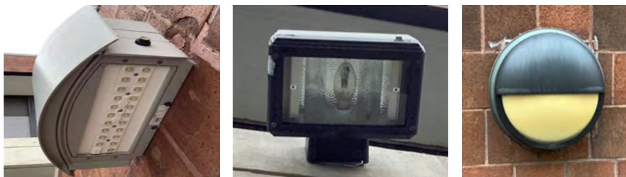
Exterior Wall Mounted LED, Metal Halide & CFL Fixtures
