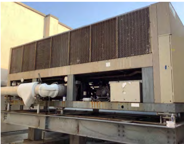
McQuay Air Cooled Screw Chiller
