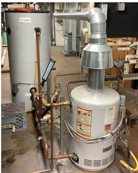
Domestic Storage Tank Water Heater
