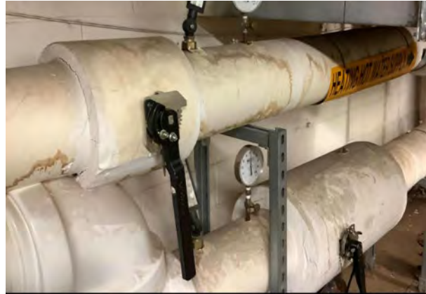
Steam to Hot Water Heat Exchanger
