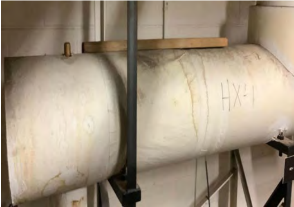
Steam to Hot Water Heat Exchanger
