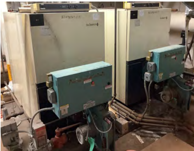
Hot Water Boilers (Back-up)
