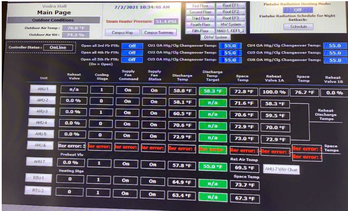
Building Energy Management System for Vodra Hall
