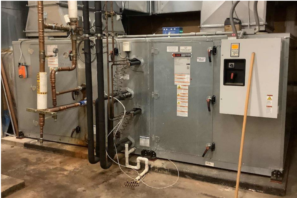
Air Handling Unit
