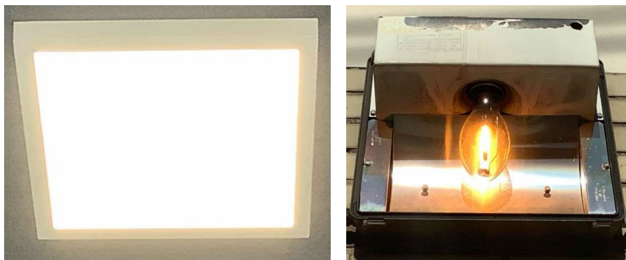
Exterior LED & HPS Fixtures
