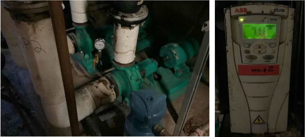
Heating Hot Water Pumps & VFD
