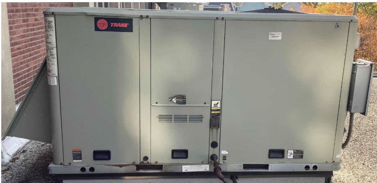
Packaged Rooftop Unit
