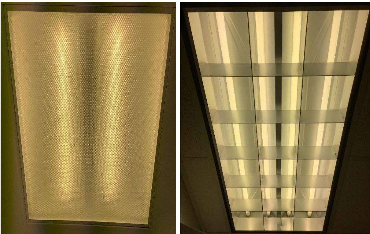
Fluorescent T8 Fixtures
