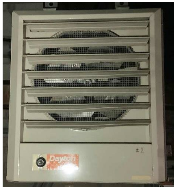
Electric Resistance Heaters
