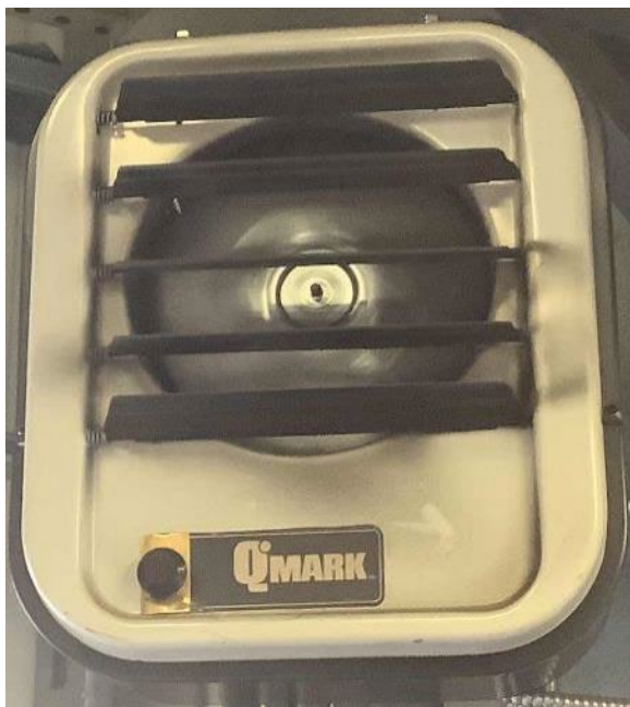
Electric Resistance Heaters
