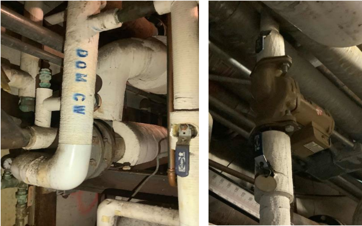
Heat Exchanger & Circulation Pump
