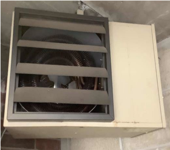
Electric Resistance Heaters
