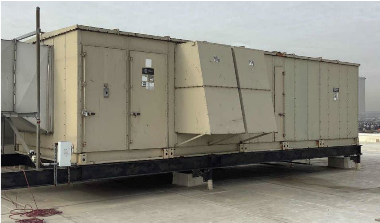
Air Handling Unit
