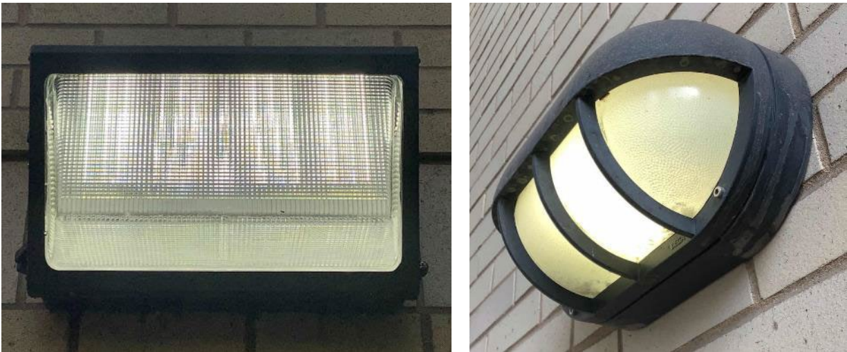
Exterior LED & MH Fixtures
