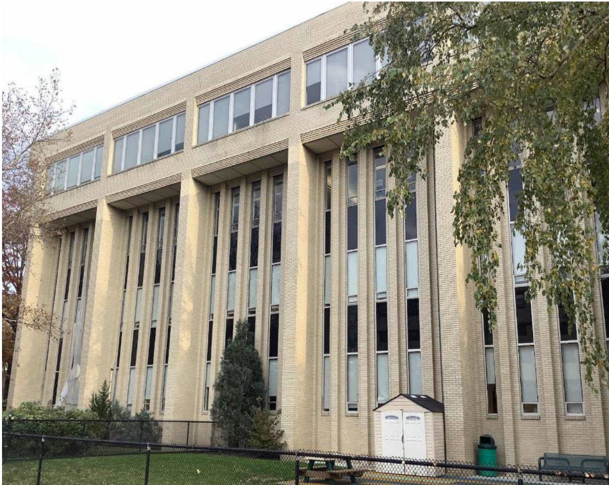
Building Walls & Windows
