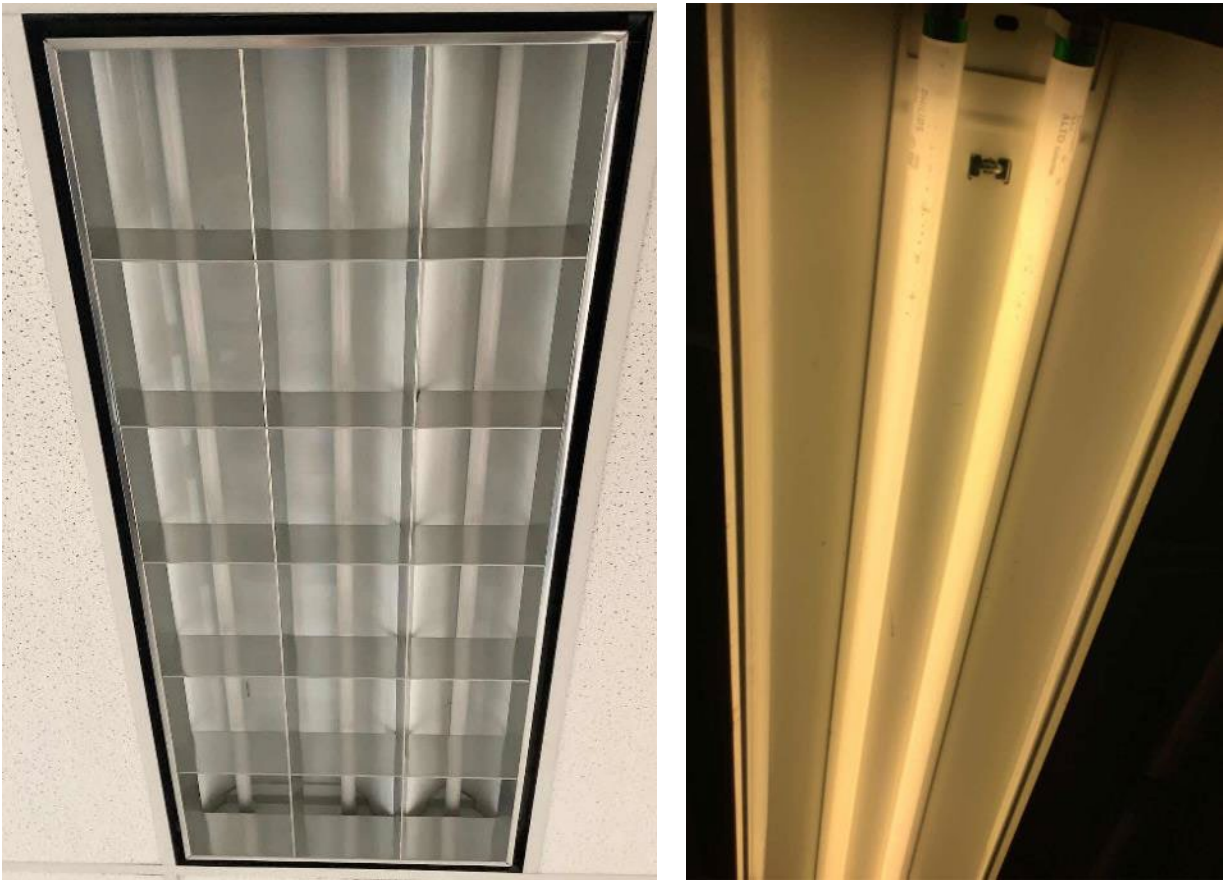
Fluorescent T8 Fixtures
