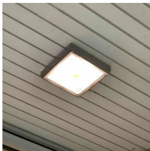
Exterior Fixture with LED Lamps
