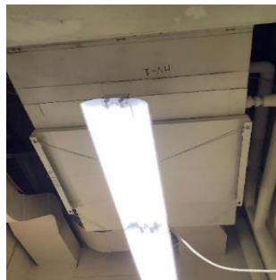
Air Handling Unit
