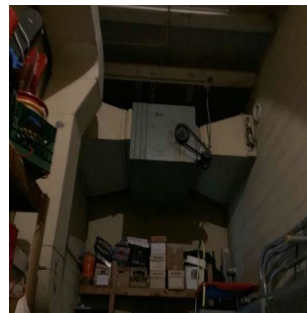
Air Handling Unit
