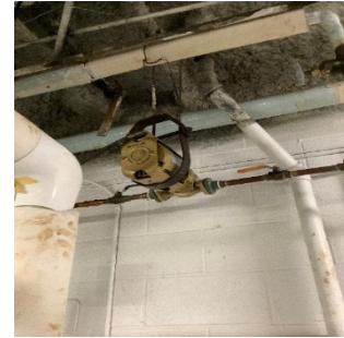
DHW Circulation Pump
