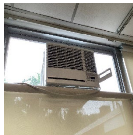
1.54 Ton Conference Room Window AC
