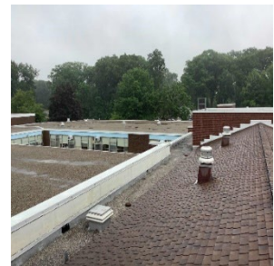
Gravel and Asphalt Roof
