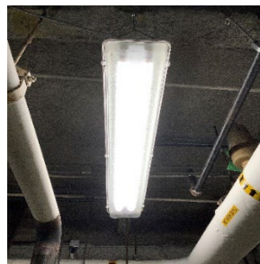
Mechanical Room LED Lighting
