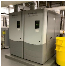
Aerco HHW Boilers
