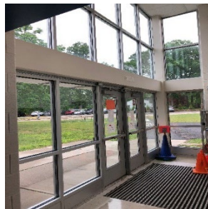
Main Entrance Doors
