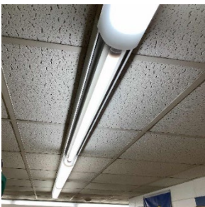
Corridor LED Lighting
