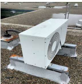
Office Heat Pump Unit
