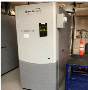
Aerco HHW Boiler
