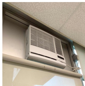
Classroom Window AC
