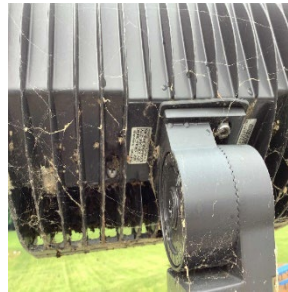
Exterior LED Flood Lamp
