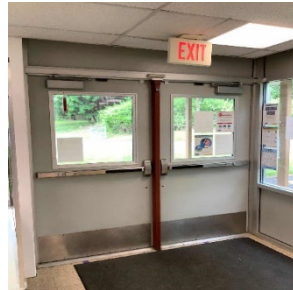
Main Entry Doors
