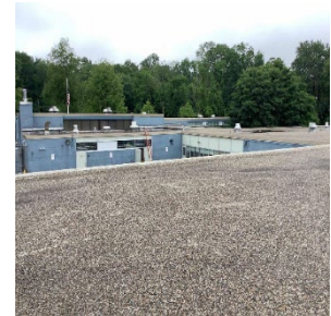
Gravel and Asphalt Roof
