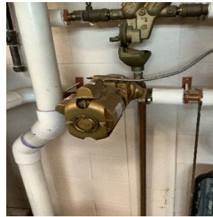
DHW Circulation Pump
