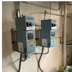
HHW Pump VFDs
