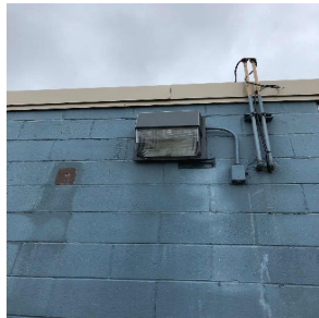
Exterior LED ED37 Lamp
