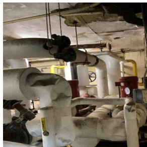
Heating Hot Water Pump
