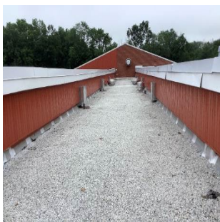
Roof – Gravel Layer
