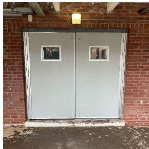
Exterior LED Lamp Fixtures
