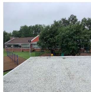
Roof – Inclined Asphalt Shingles
