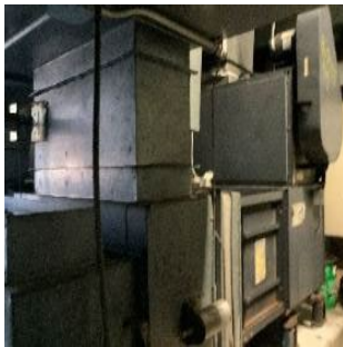
Air Handling Units
