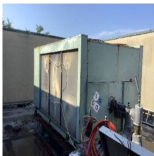
Chiller on Roof
