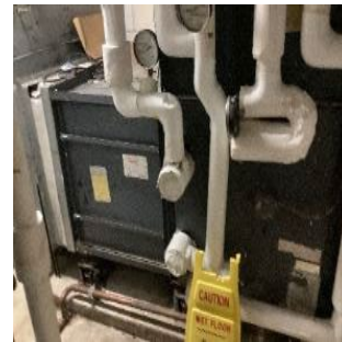
Air Handling Units
