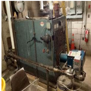
Hot Water Boiler
