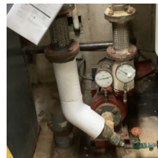
Chilled Water Circulation Pump
