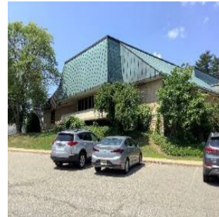
Exterior and Standing Seam Roof
