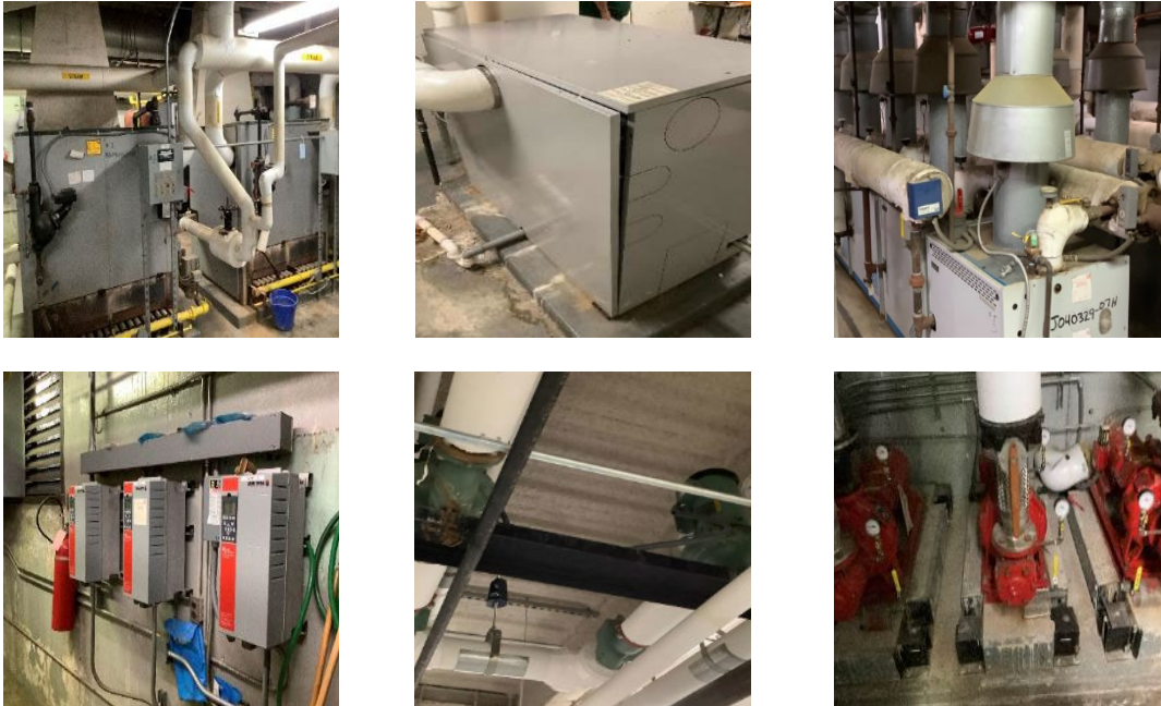
Steam Boilers, Hot Water Boilers, VFDs, Hot Water Pumps
