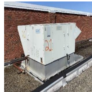
Rooftop Packaged Unit
