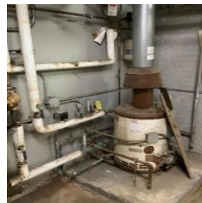
Hot Water Boiler
