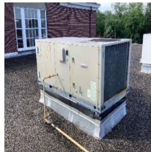
Rooftop Packaged Unit
