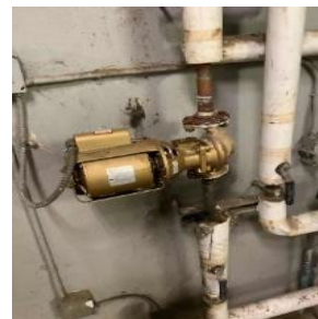
DHW Circulation Pump
