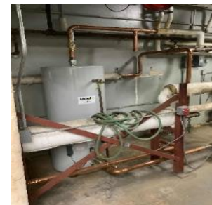
Hot Water Storage Tank
