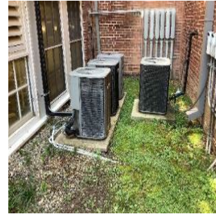
Condensing Units for Split System Cooling Equipment
