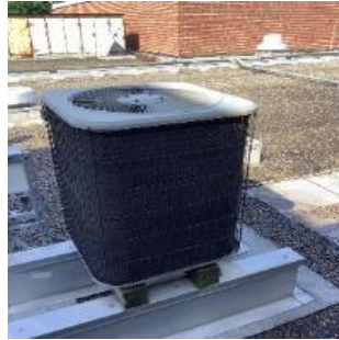
Condensing Units for Split System Cooling Equipment
