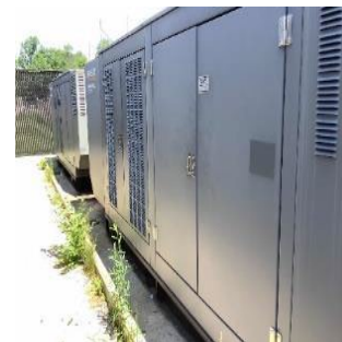
Back-up Diesel Generator
