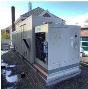
Rooftop Packaged Unit
