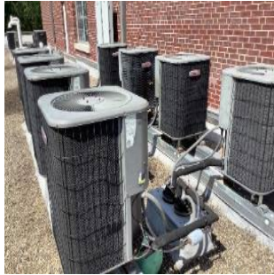
Condensing Units for Split System Cooling Equipment
