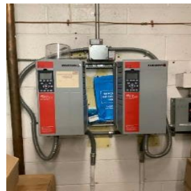
HHW Pump VFDs
