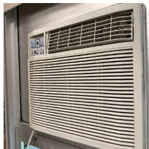
Classroom Window AC
