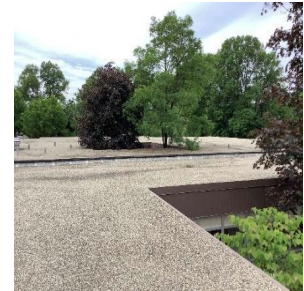
Gravel and Asphalt Roof
