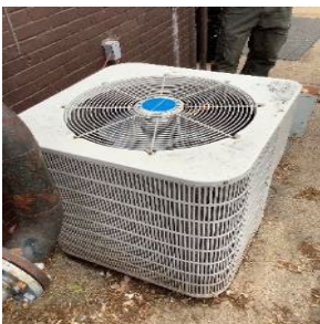
Office Condensing Unit
