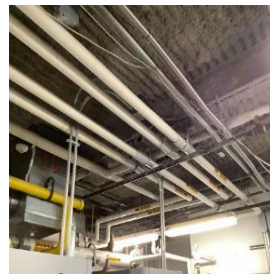
HHW Pipe Insulation
