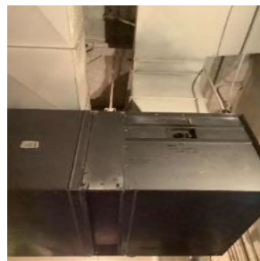
Gymnasium/Multipurpose Air Handling Unit
