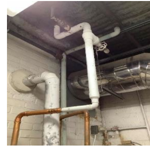
Uninsulated DHW Piping
