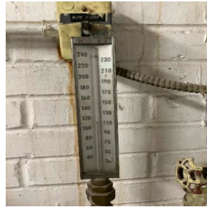
DHW Supply Temperature
