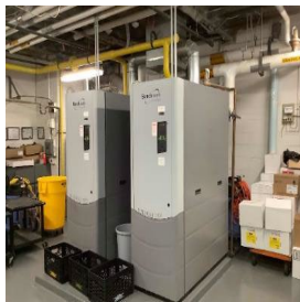
Aerco HHW Boilers
