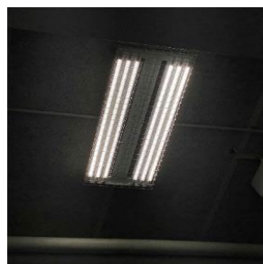
Gym/ Multipurpose Fixture
