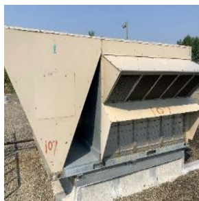
Media Center RTU
