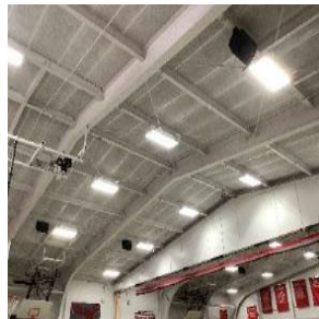
Gymnasium High Bay
