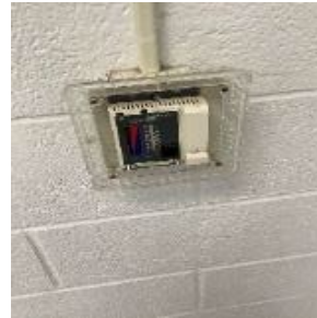
Local Temperature Controls
