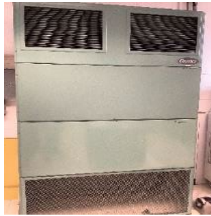
Server Room AHU
