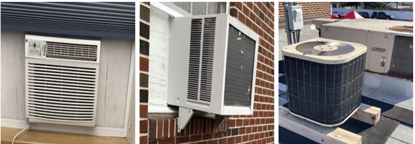
Typical Window ACs & Condensing Unit
