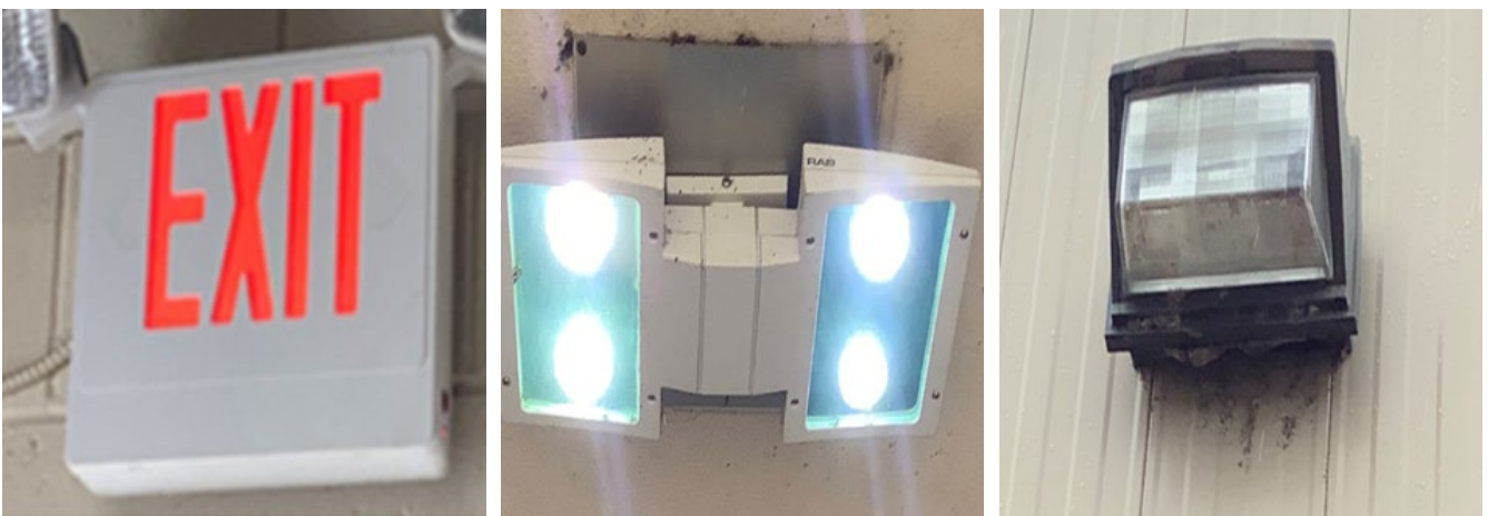
LED Exit Sign, Recessed, and Wall Mounted Exterior LED Fixtures
