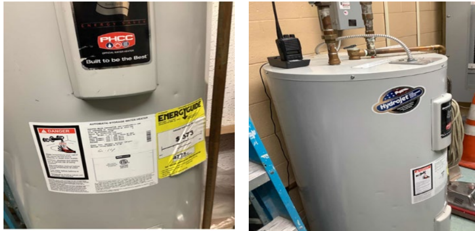
Storage Tank Water Heater
