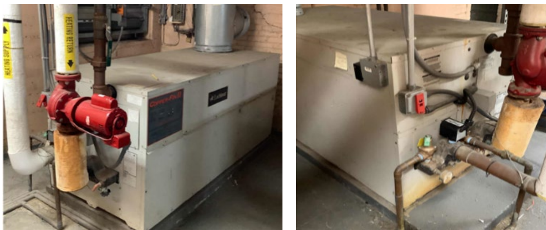
Lochinvar Non-Condensing Boilers
