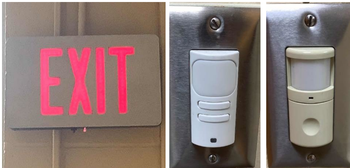
LED Fixtures & Occupancy Sensors
