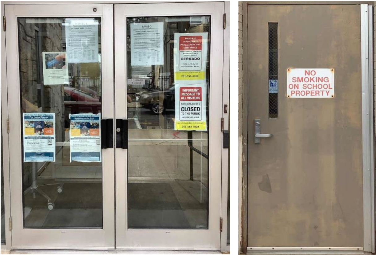
Entrance & Exit Doors
