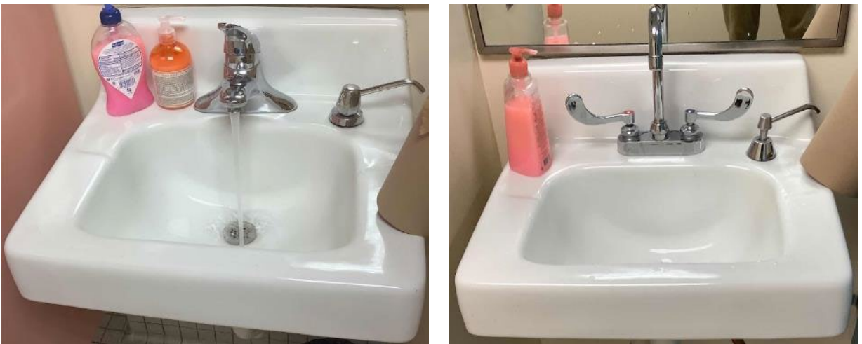
Typical Restroom Sinks
