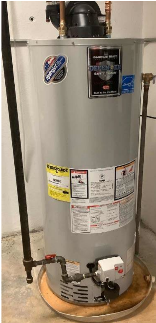
Gas-fired Storage Tank Water Heater
