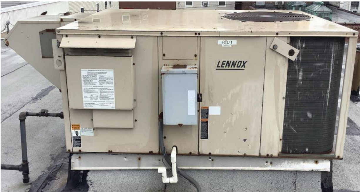
Rooftop Unit RTU-1
