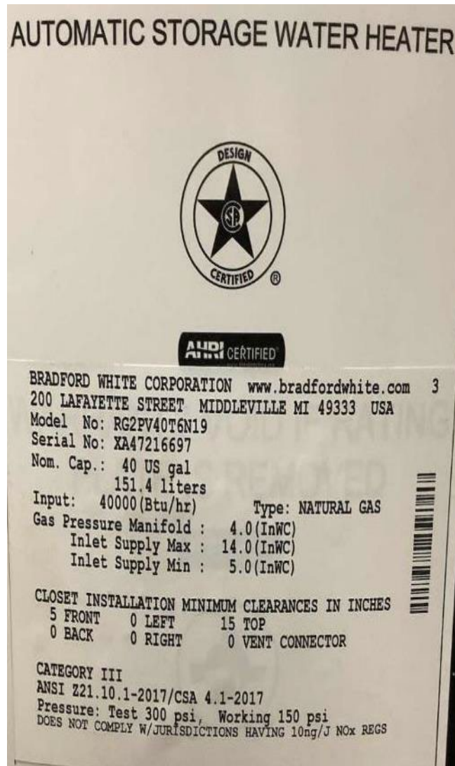
Gas-fired Storage Tank Water Heater
