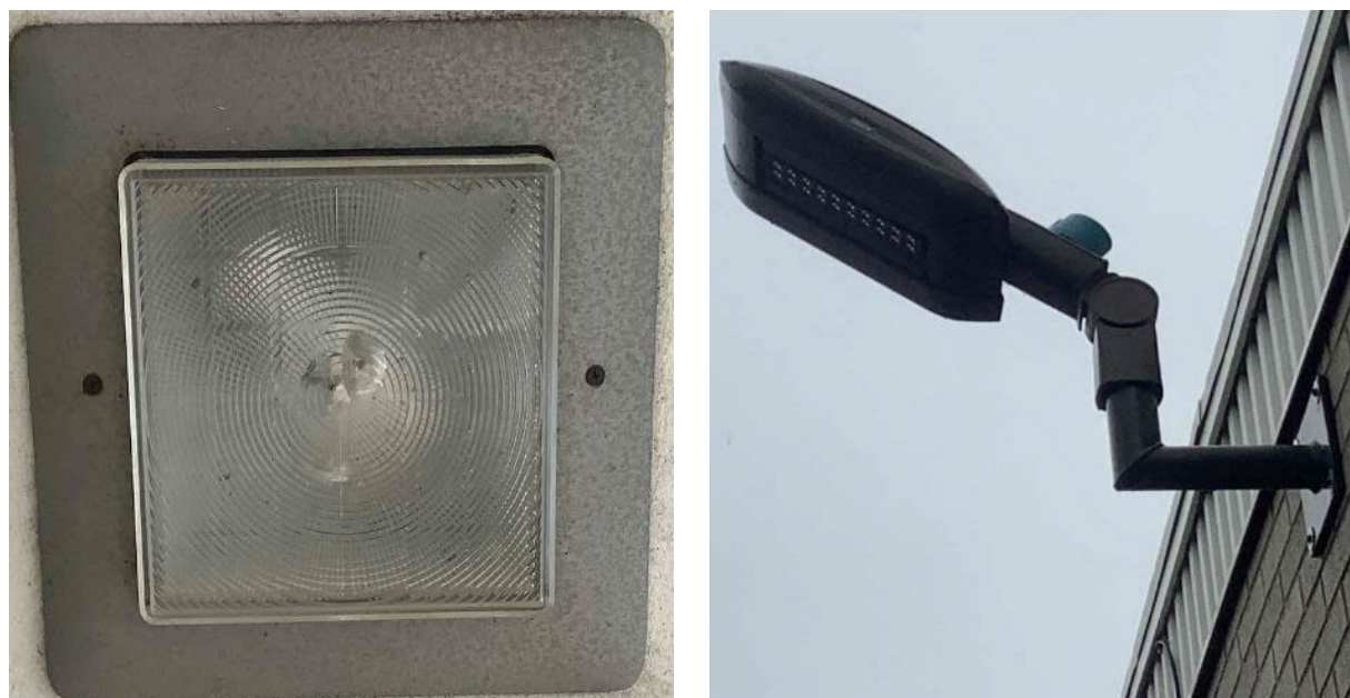
Exterior CFL & LED Fixtures
