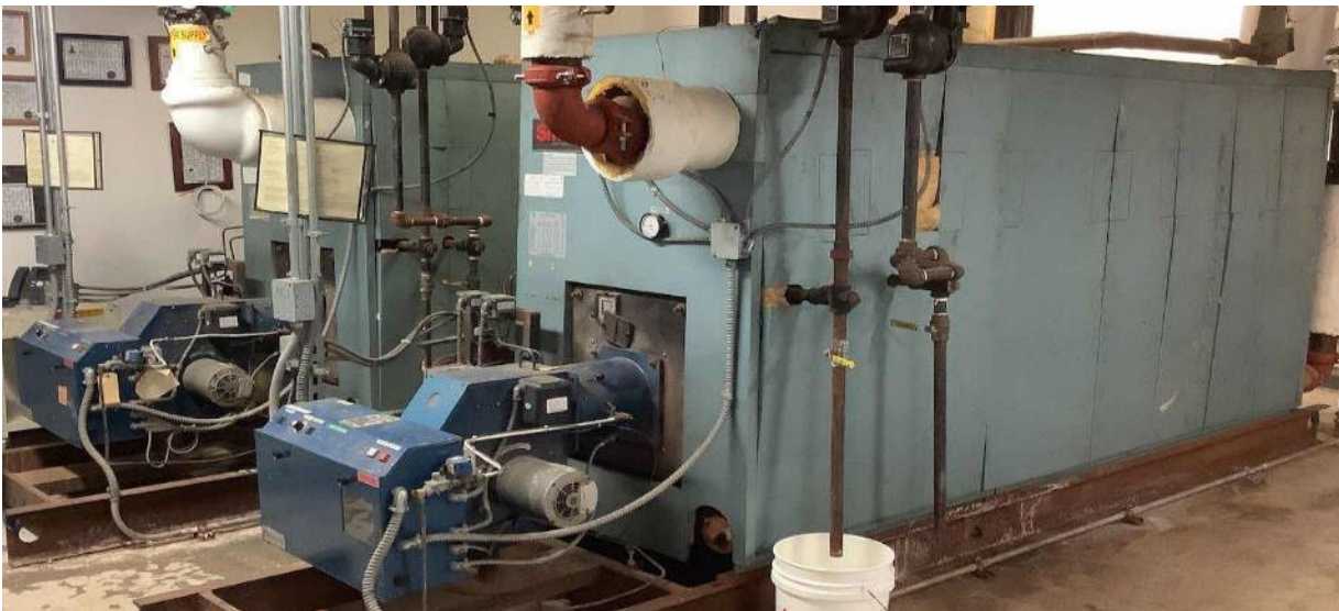
Hot Water Boilers
