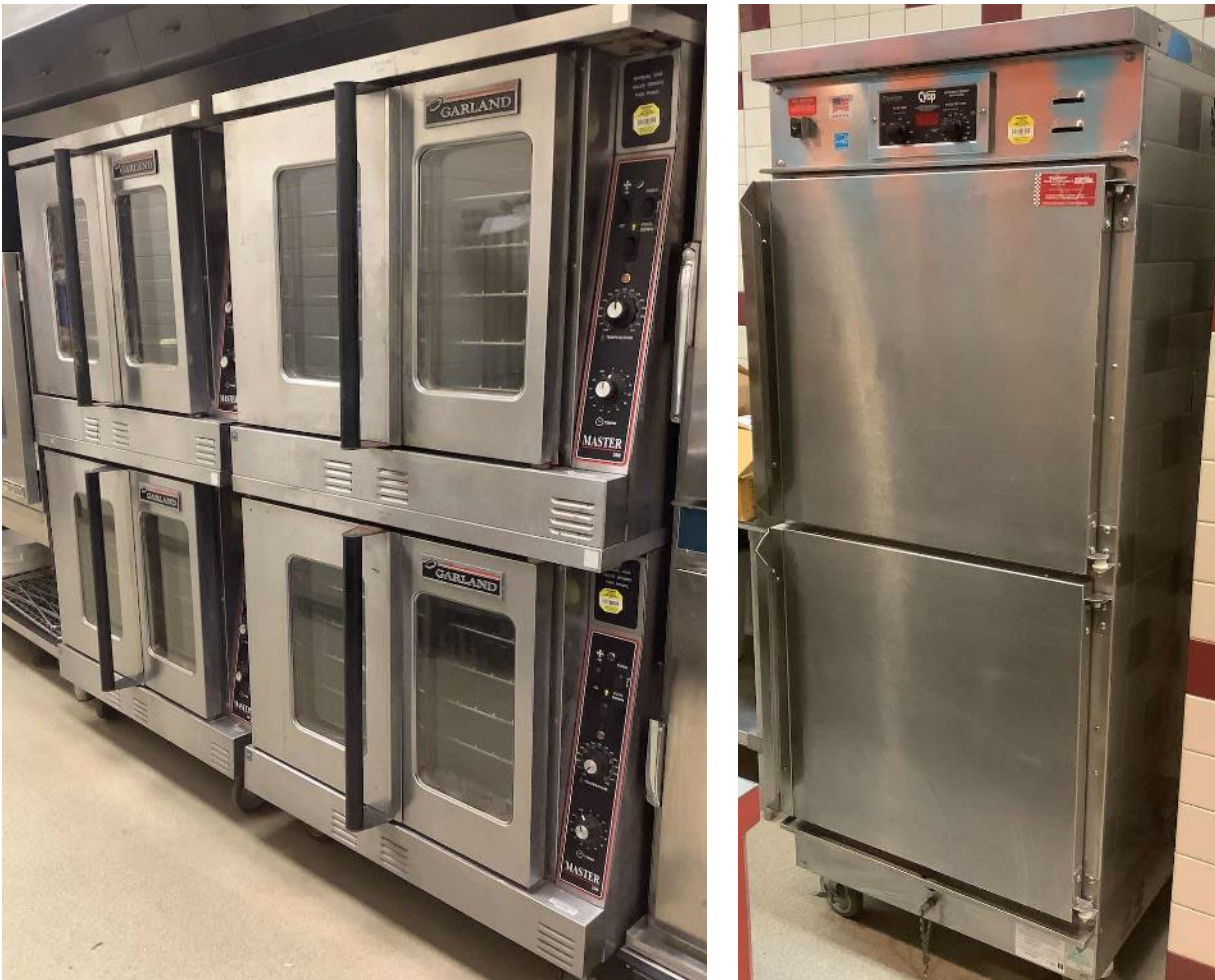
Gas-fired Convection Ovens & Electric Holding Cabinet
