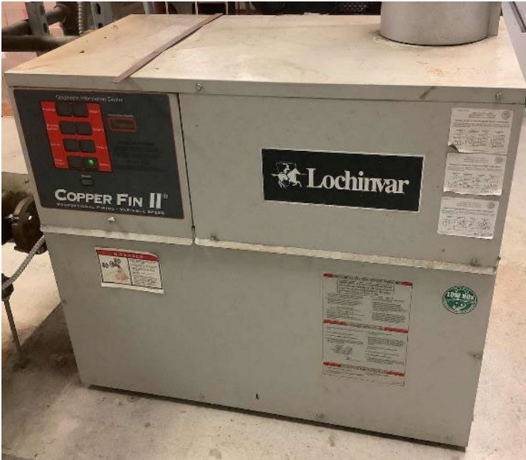
Gas-fired Domestic Hot Water (DHW) Boiler & Circulation Pump
