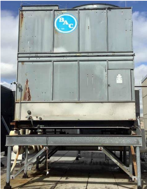
Cooling Tower & Condenser Water Pumps (CWP-8 & CWP-9)
