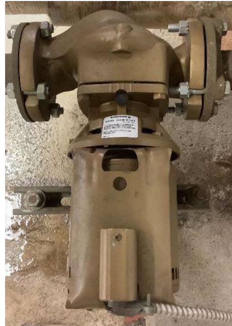
Gas-fired Domestic Hot Water (DHW) Boiler & Circulation Pump
