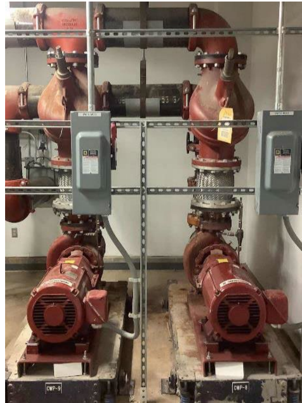
Cooling Tower & Condenser Water Pumps (CWP-8 & CWP-9)
