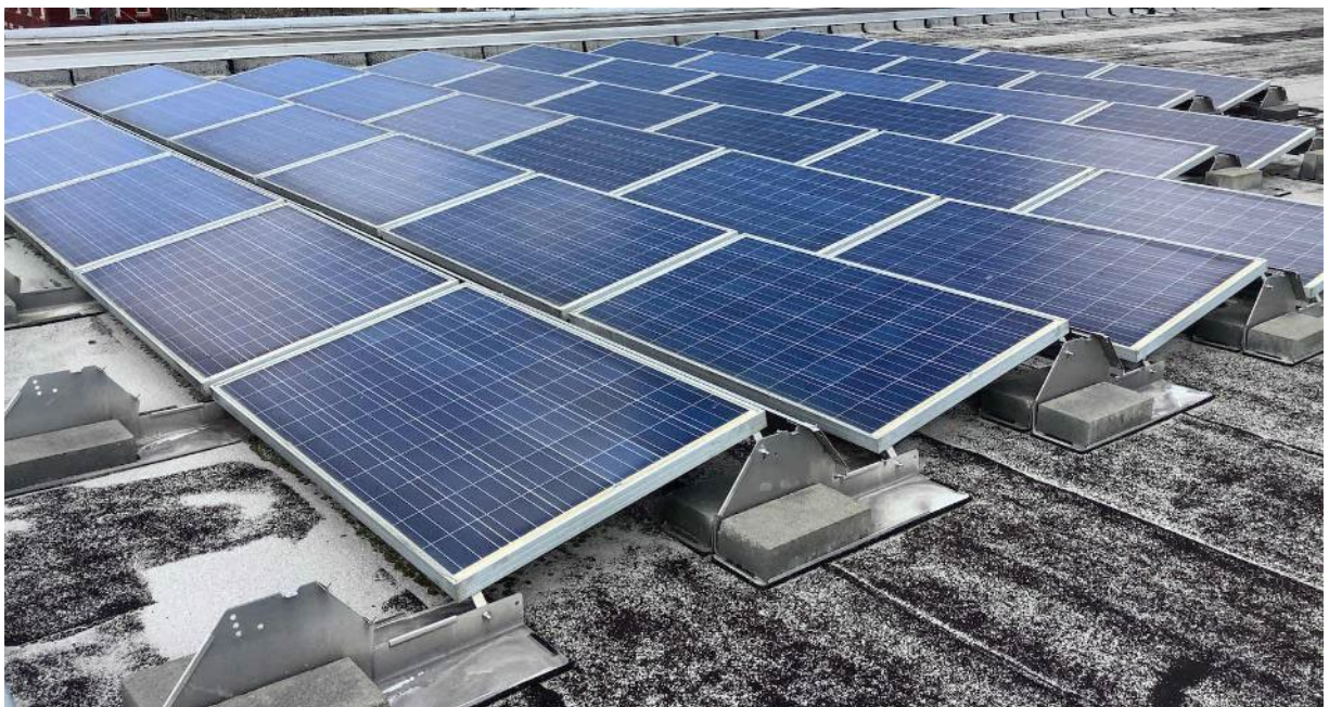
Rooftop Solar Panels
