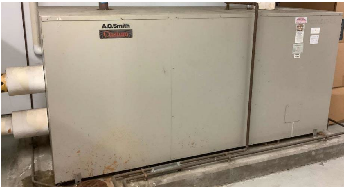
DHW Storage Tank
