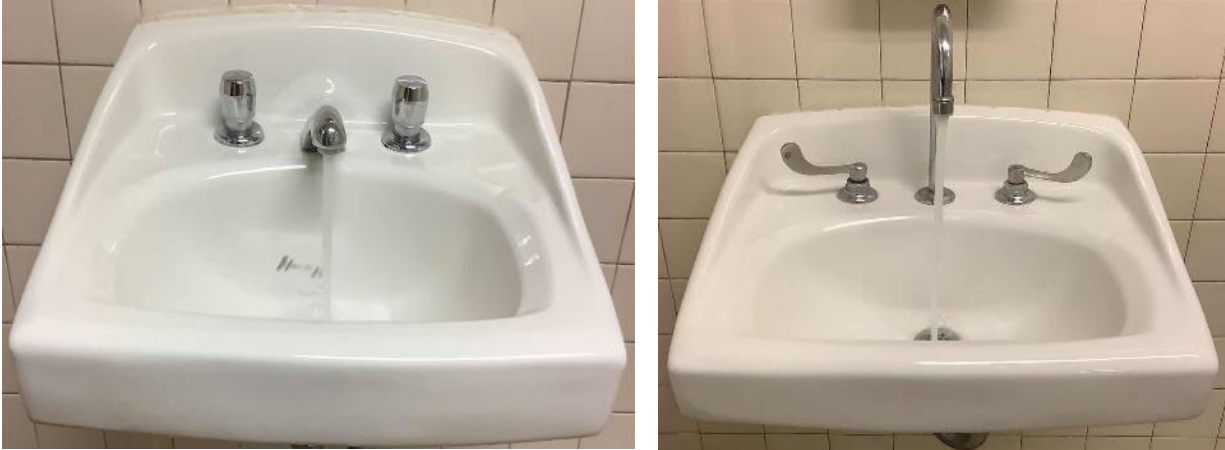
Typical Restroom Sinks
