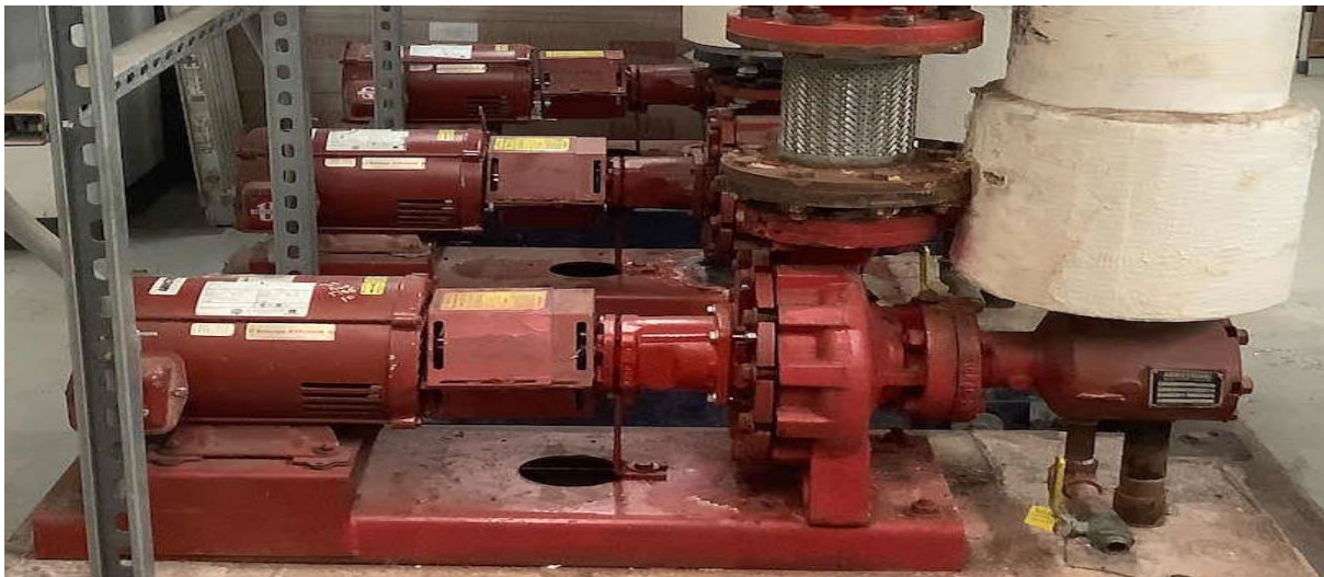
Heating Hot Water Pumps
