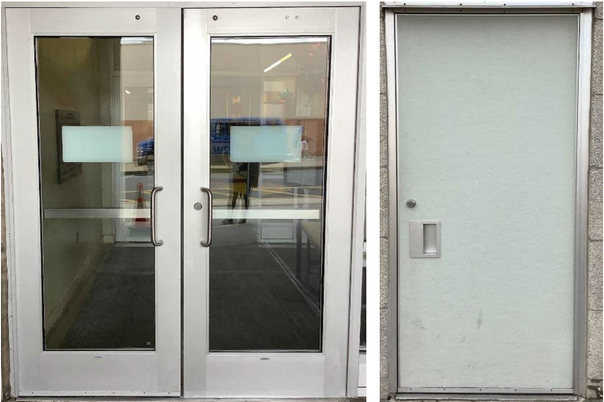
Entrance & Exit Doors
