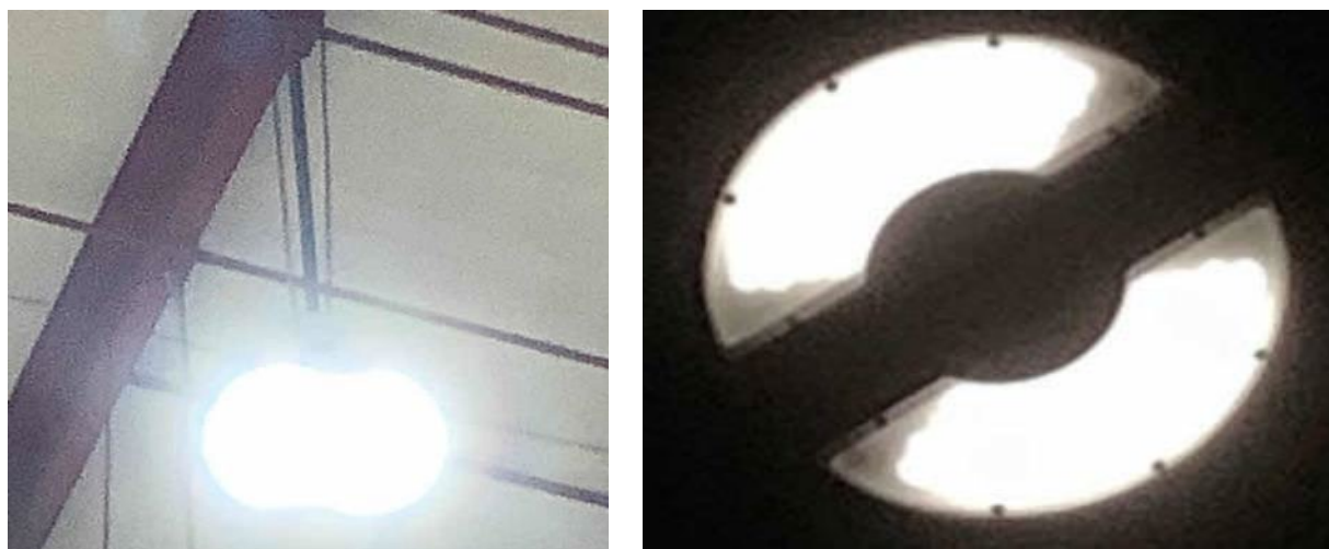
Gymnasium High Bay LED Fixtures
