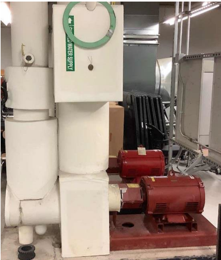
Chilled Water Pumps (CHWP-6 & CHWP-7) & VFD
