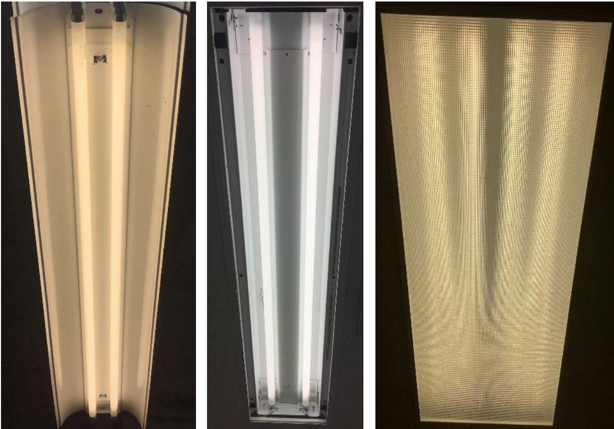
Fluorescent T8 Fixtures
