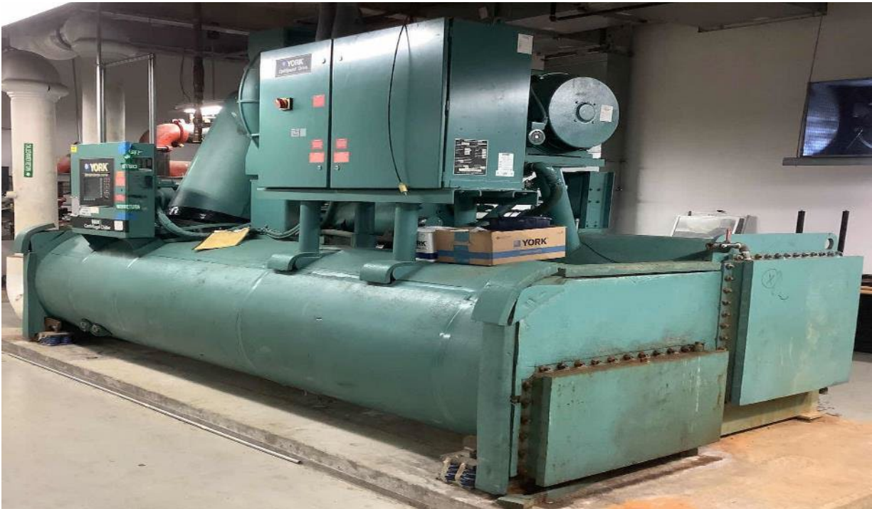
Air Cooled Chiller
