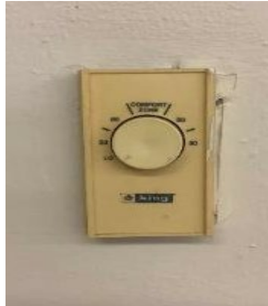
Manual thermostats - Classrooms
