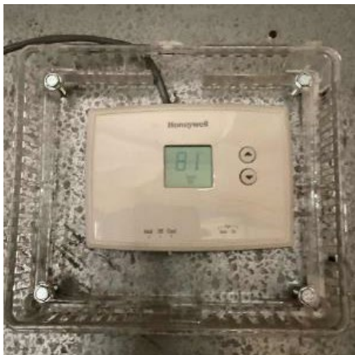
Programmable thermostats - Gymnasium
