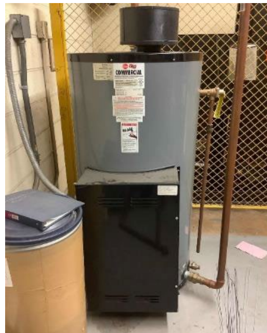
Electric water heater – Elevator room
