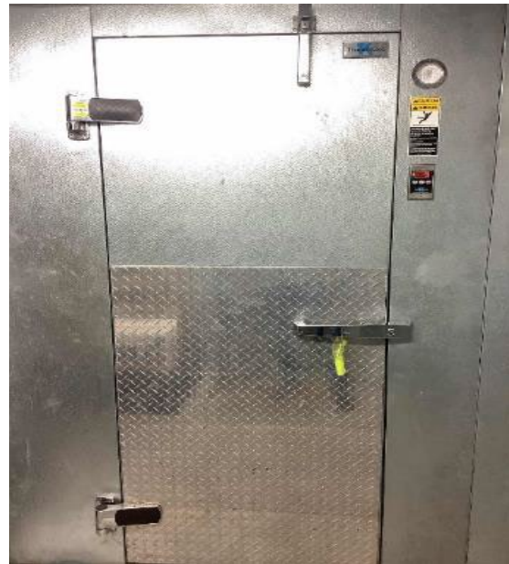
Walk-in medium temperature freezer
