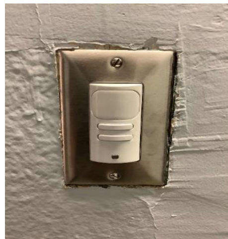
Occupancy Sensor - Restroom
