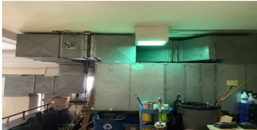
Air handling unit - Gymnasium
