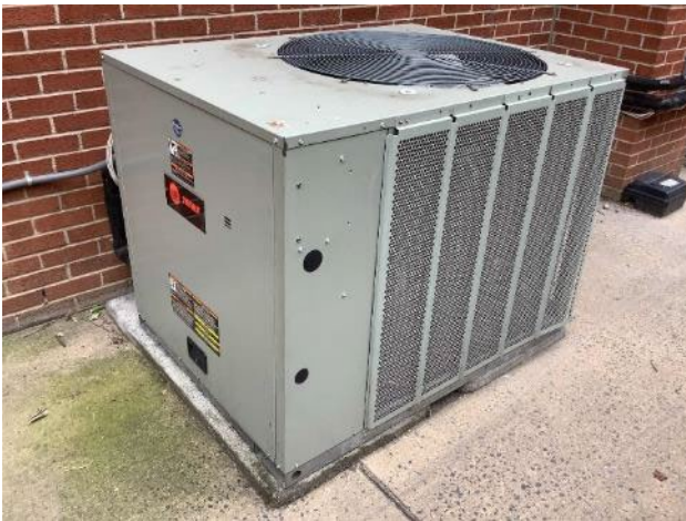
Heat pump Condenser– Cafeteria/Kitchen
