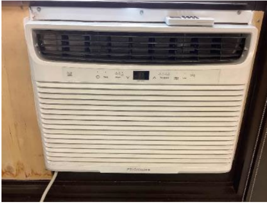
Window AC - Classroom
