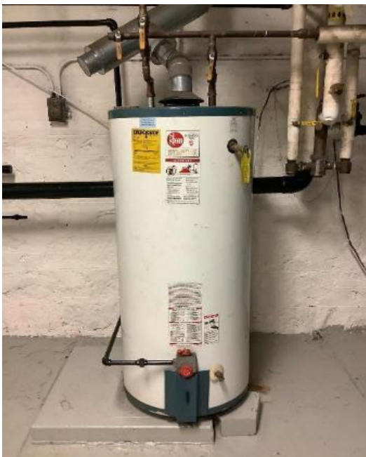
Gas-fired Domestic Water Heater (DHW) – Boiler room
