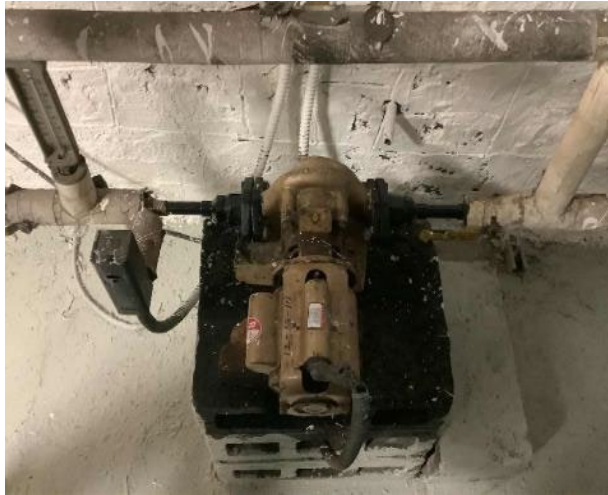
Fuel oil pump
