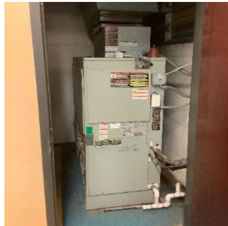
Heat pump – Cafeteria/Kitchen
