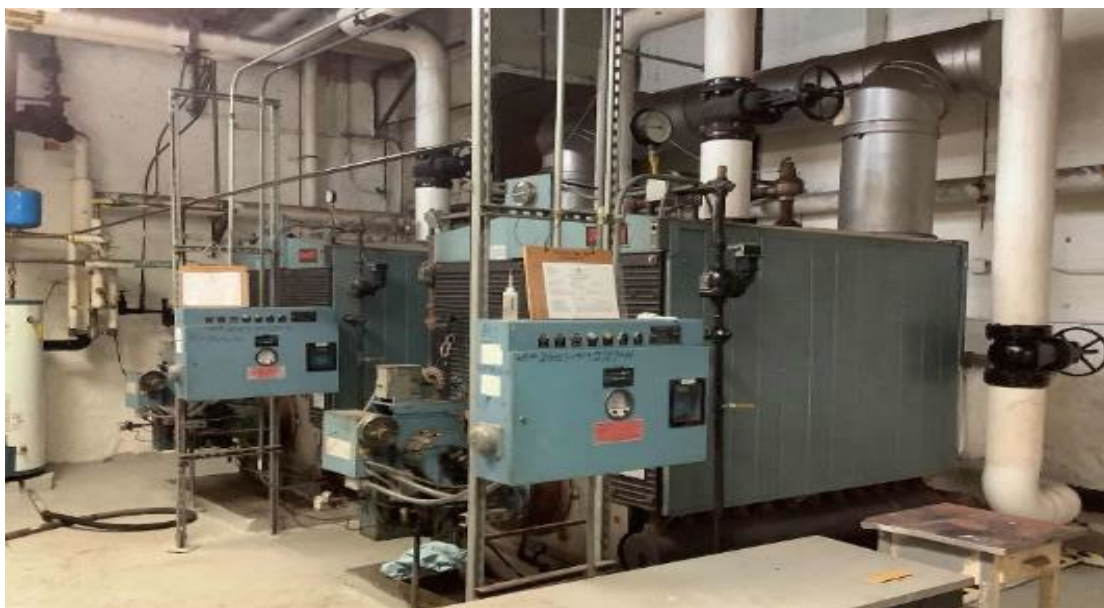
Non-condensing boilers
