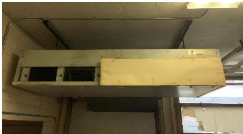
Fan coil unit - Classroom
