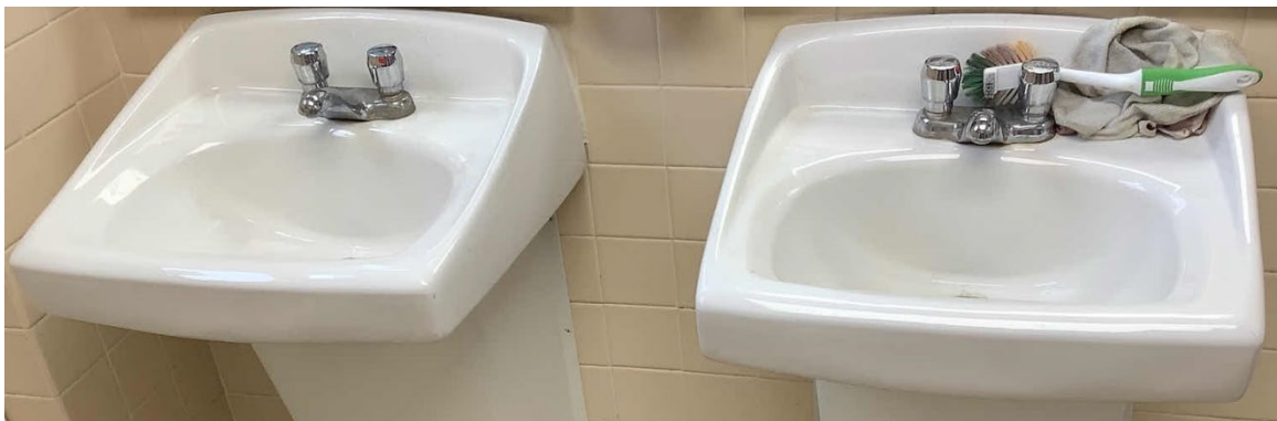
Typical restroom sinks
