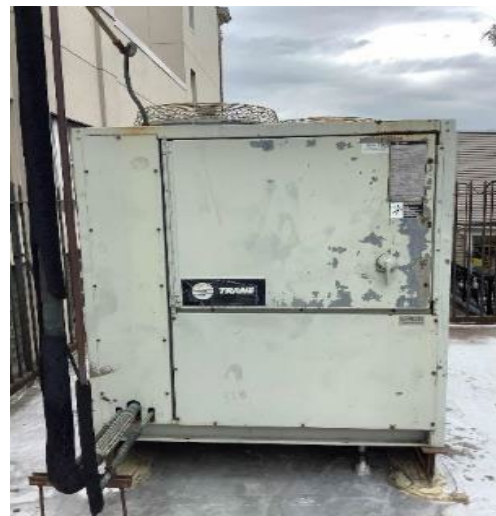
Gymnasium condensing unit
