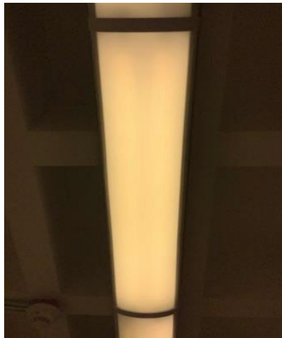
40W surface mounted interior LED fixtures
