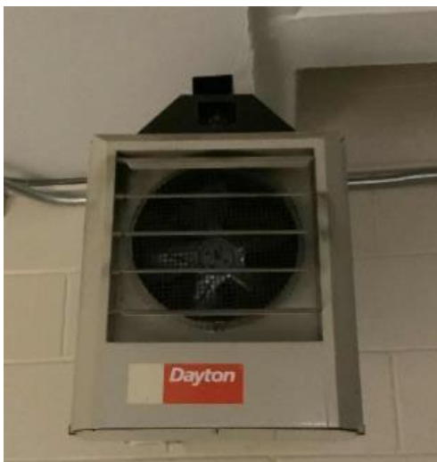
Electric resistance heater
