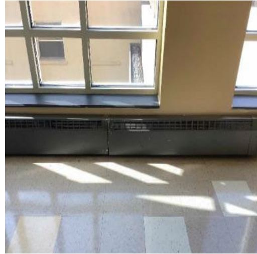
Hot water baseboard (corridor)
