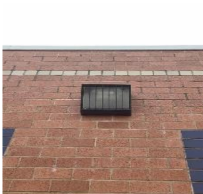
Exterior wall pack - 100W MH fixture
