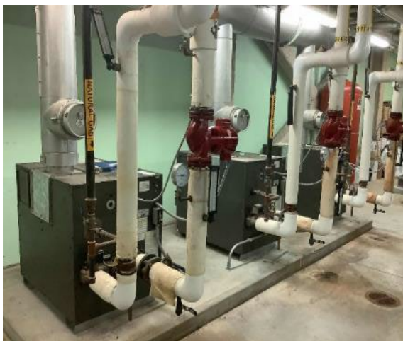
Non-condensing hot water boilers
