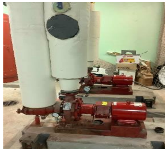
Heating hot water pumps
