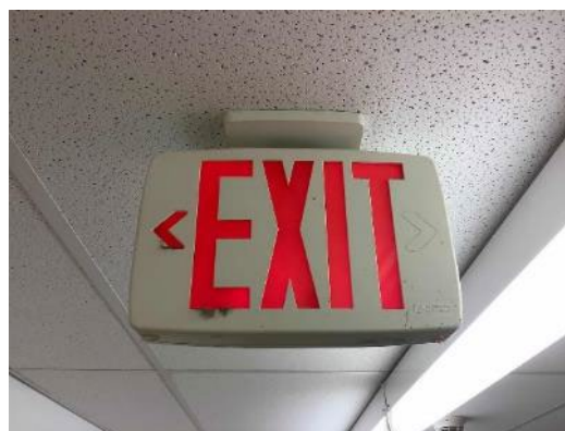
2W LED Exit signs
