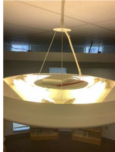
CFL fixtures - Library
