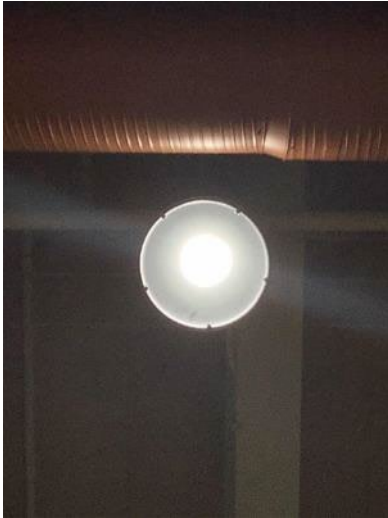
100W high bay LED fixtures - Gymnasium
