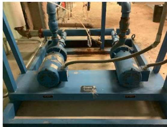
DHW booster pumps
