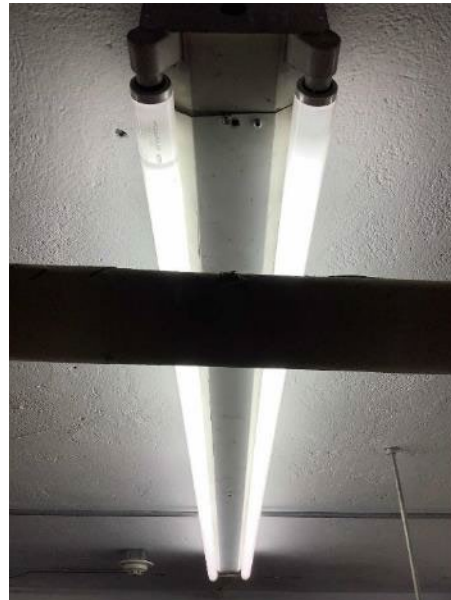
8-foot T12 fixture - Storage
