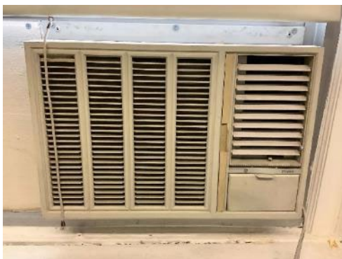
Older Window AC unit
