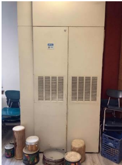
Unit ventilators - Classroom
