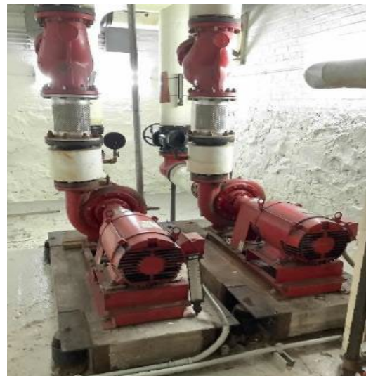
Hot water pumps
