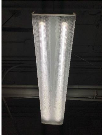
Boiler room – LED linear tube
