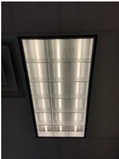
Typical Classroom – 4 foot T8 fixture
