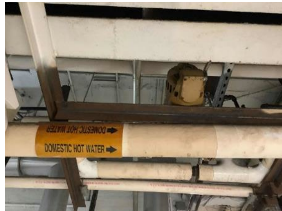
DHW circulation pumps
