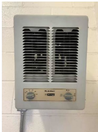
Electric resistance heater
