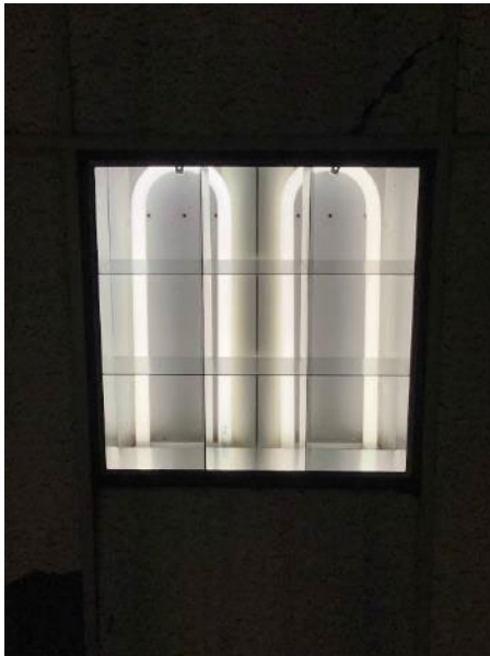
2-foot U bend T8 fixture - Stairwell
