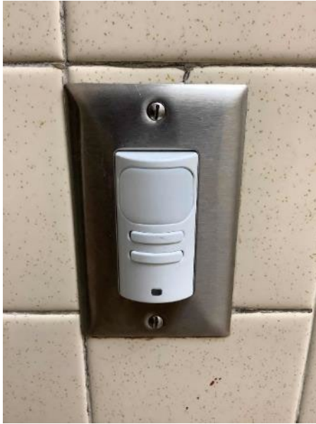
Occupancy sensors - Restroom
