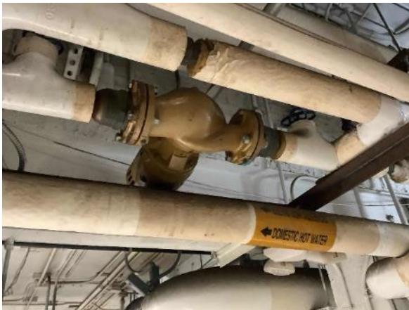
DHW circulation pumps
