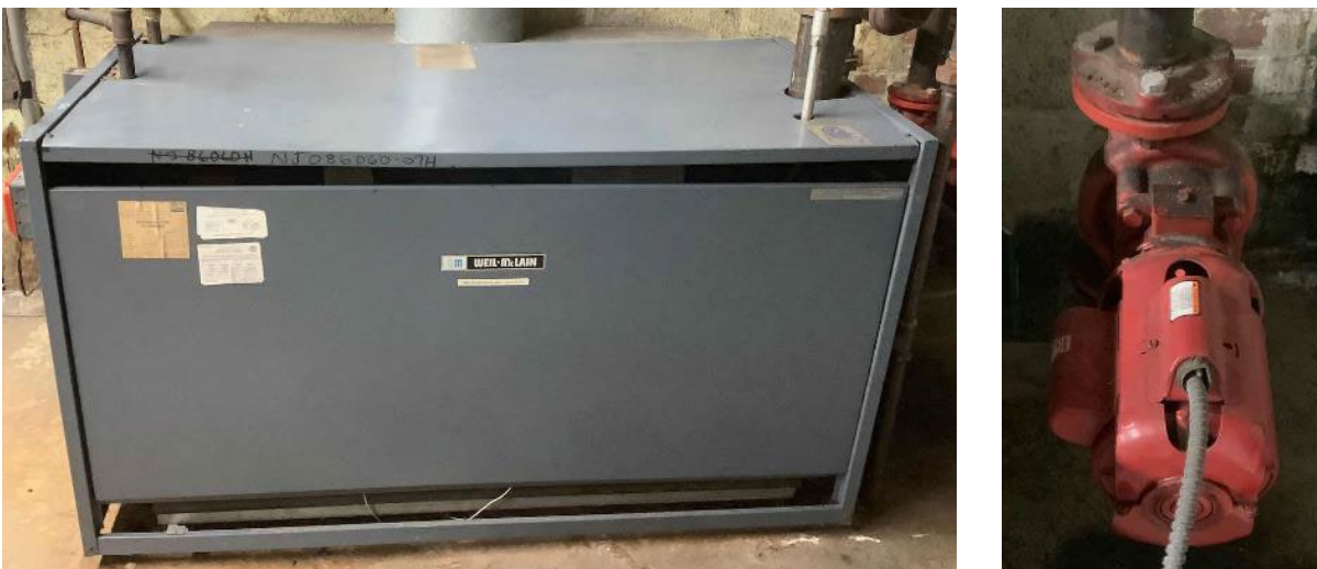
Hot Water Boiler & Heating Hot Water Pump
