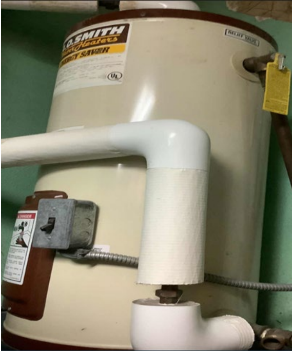
Gymnasium (Electric) Storage Tank Water Heaters
