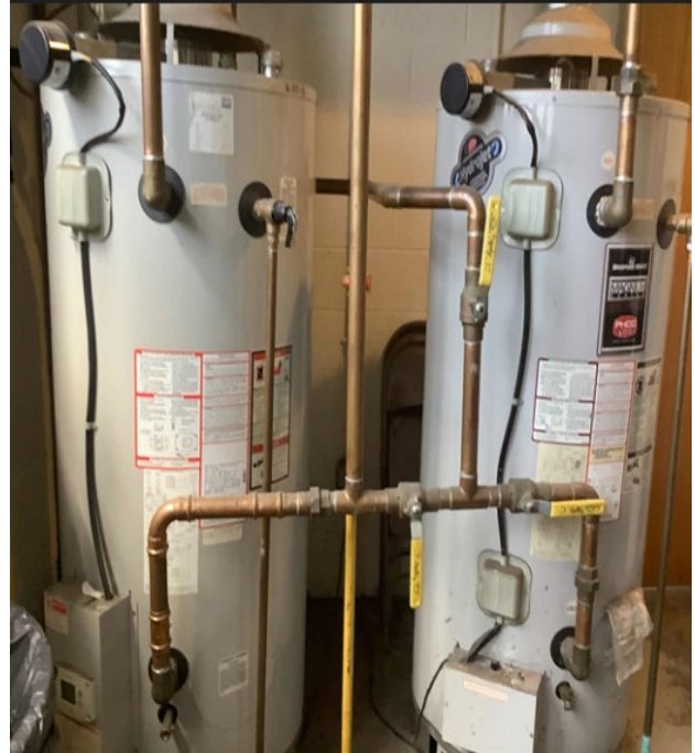
Multipurpose Room (Gas) Storage Tank Water Heaters
