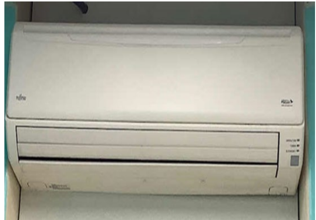
Split System Air Source Heat Pump Unit
