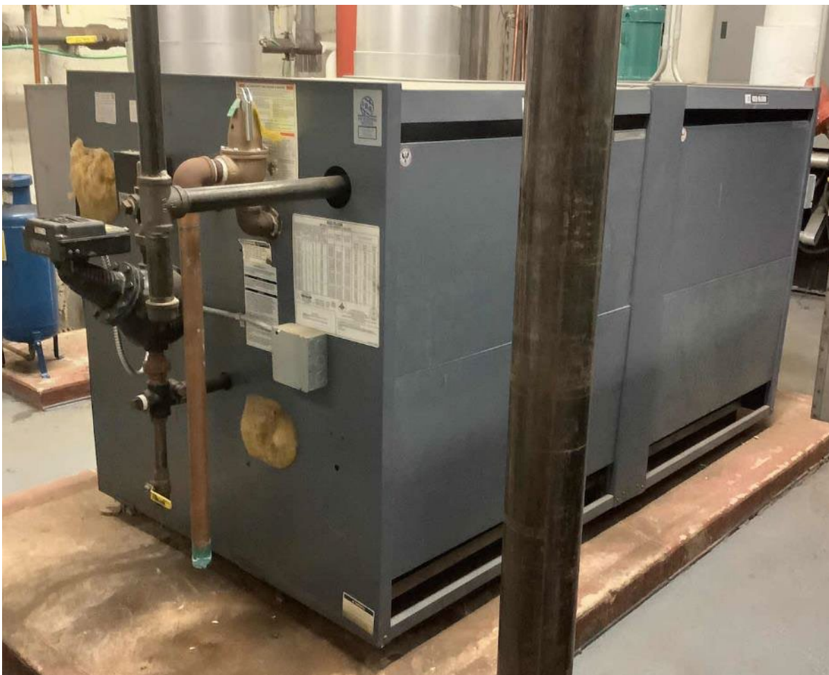
Hot Water Boiler
