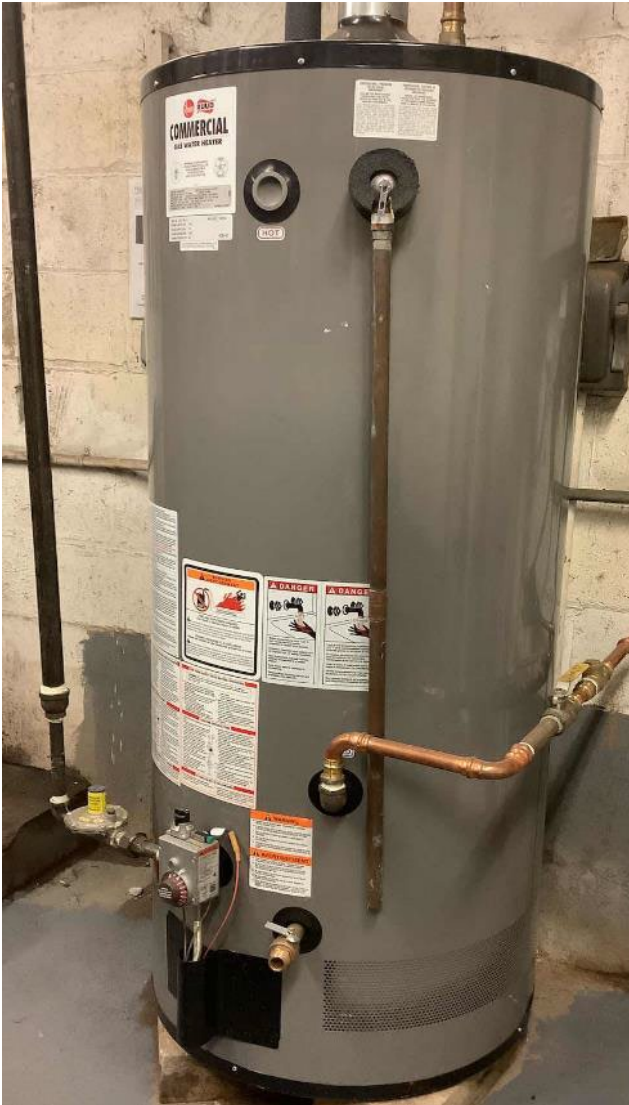
Water Heater & Circulation Pump
