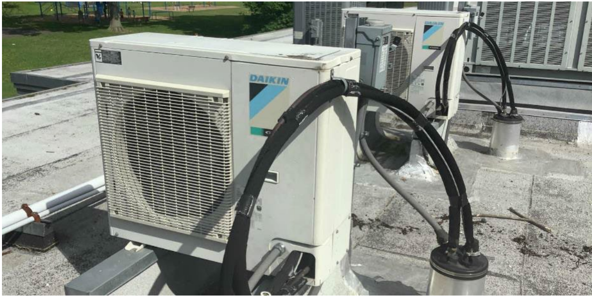
Mini-split Heat Pump Units
