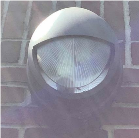
Exterior CFL & HPS Fixtures
