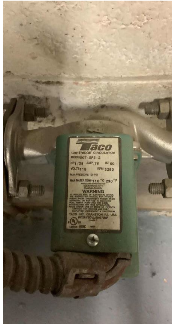
Water Heater & Circulation Pump
