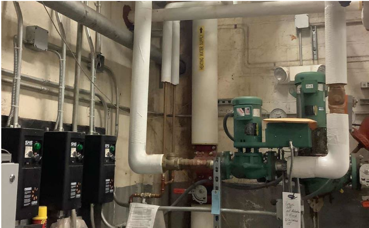
Heating Hot Water Pumps
