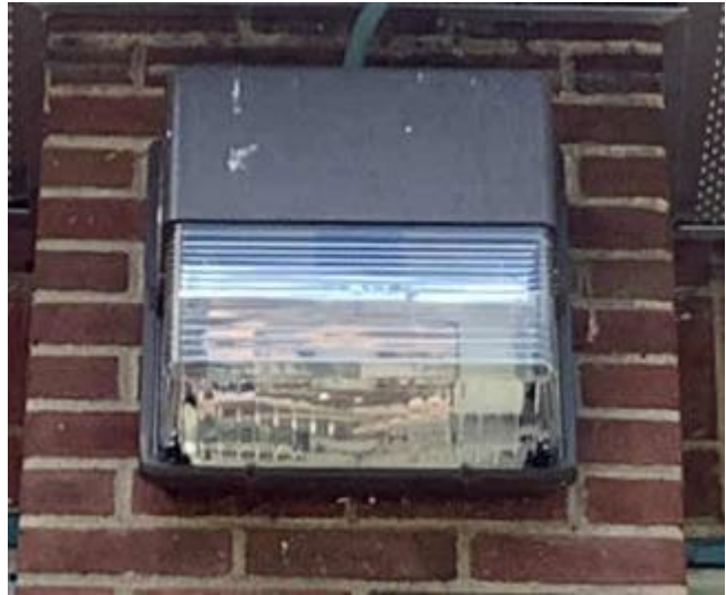
Exterior CFL & HPS Fixtures
