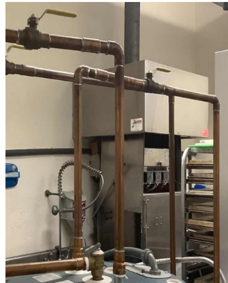
Kitchen Electric Storage Tank Water Heaters & Insulated Hot Water Pipes
