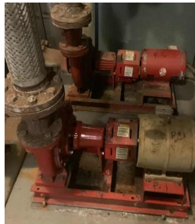
AERCO Condensing Boilers & 5 hp Hot Water Pumps
