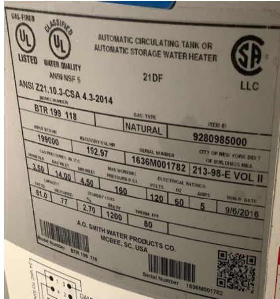
Main Gas-Fired Storage Tank Water Heater
