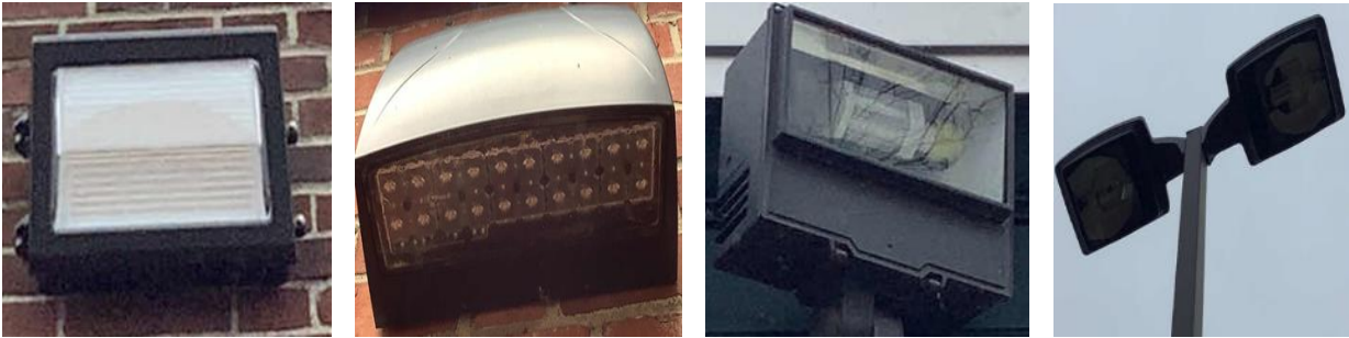
LED Fixtures, LED Corn Bulbs & Metal Halide
