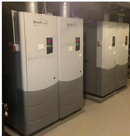
AERCO Condensing Boilers & 5 hp Hot Water Pumps
