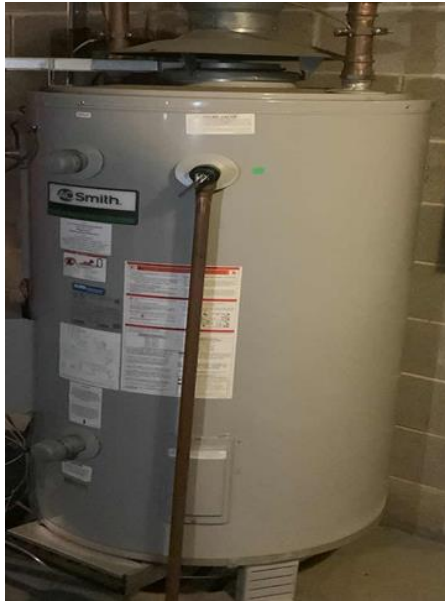
Main Gas-Fired Storage Tank Water Heater
