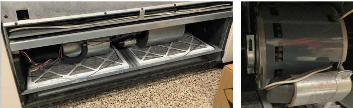
Typical Unit Ventilator
