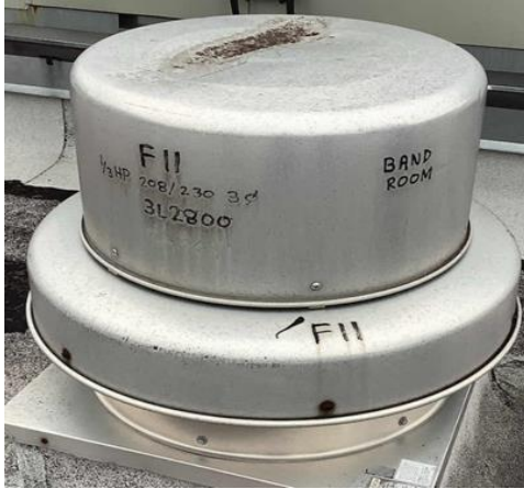
Typical General Exhaust Fan & Kitchen Hood
