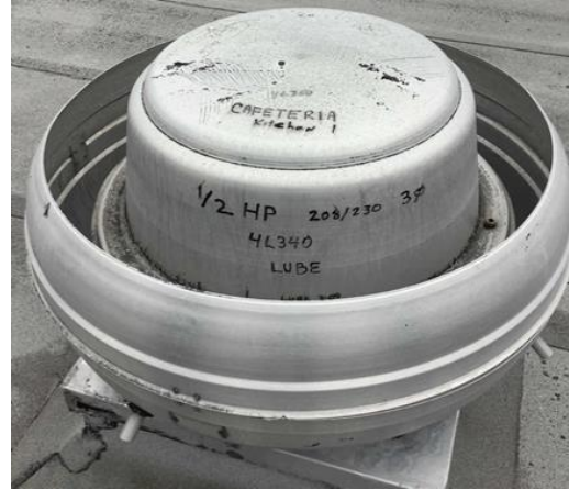
Typical General Exhaust Fan & Kitchen Hood
