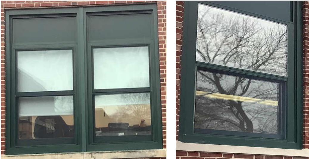
Typical Building Windows
