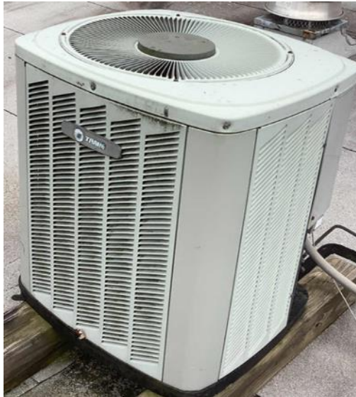
Typical Trane Condensing Unit
