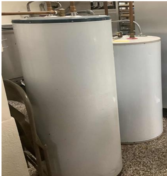
Kitchen Electric Storage Tank Water Heaters & Insulated Hot Water Pipes
