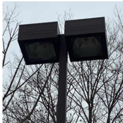
Wall & Pole Mounted Metal Halide Lamps
