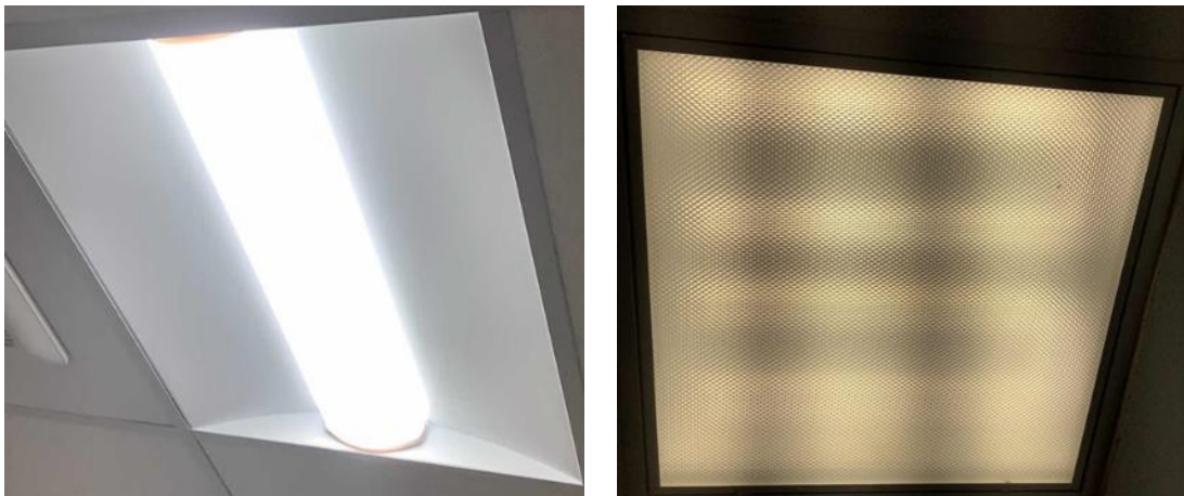
LED Fixture & LED U-Bend Tubes
