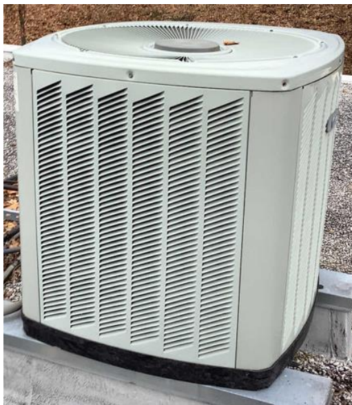
Typical Trane Condensing Unit
