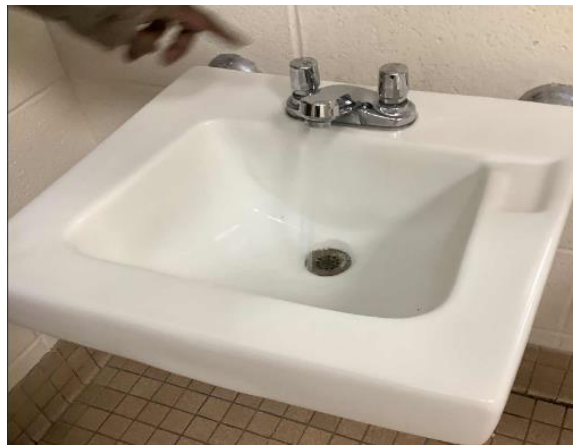
Sink with 2.2 gpm
