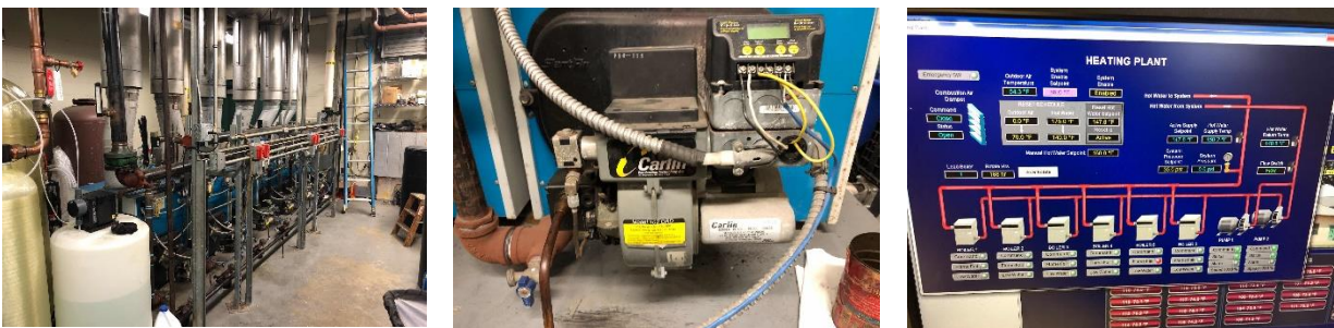
Boilers, combustion air fan, and BMS diagram
