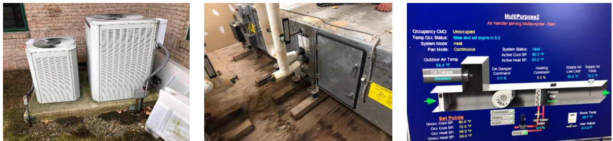
Outside condensing units, AHUs, and BMS diagram
