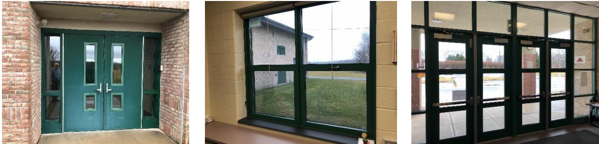
Exterior door, window, and exterior main entrance
