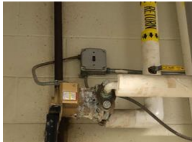
Oil fired storage water heater, DHW circulation pump, and propane-fired storage water heater
