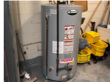
Oil fired storage water heater, DHW circulation pump, and propane-fired storage water heater
