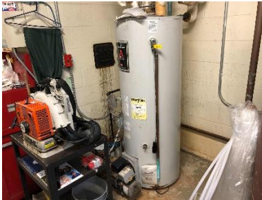
Oil fired storage water heater, DHW circulation pump, and propane-fired storage water heater
