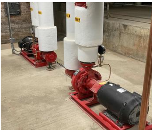
Constant Flow Hot Water Distribution Pumps & Motors
