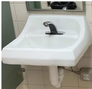
Typical Restroom Low Flow Devices
