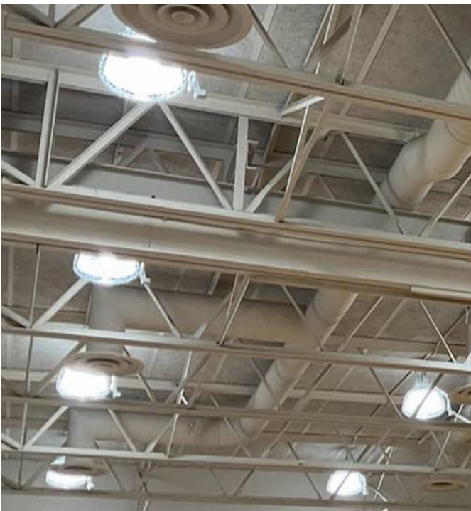
Gym LED High Bay, LED 2x2 & LED Recessed Lamps
