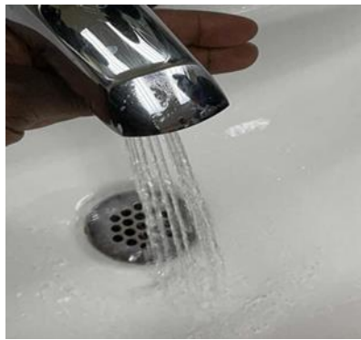
Typical Restroom Low Flow Devices
