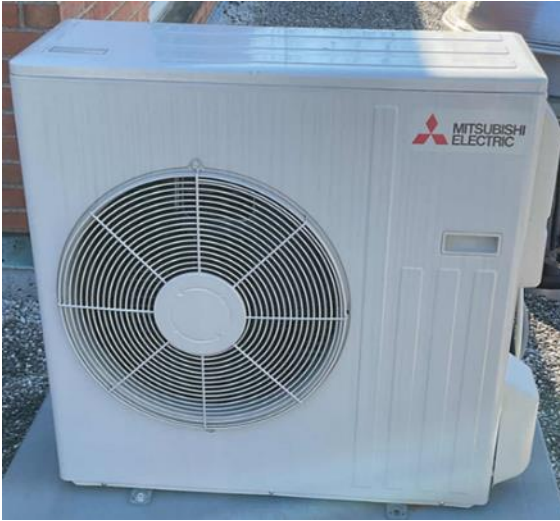
Ductless Split Systems AC
