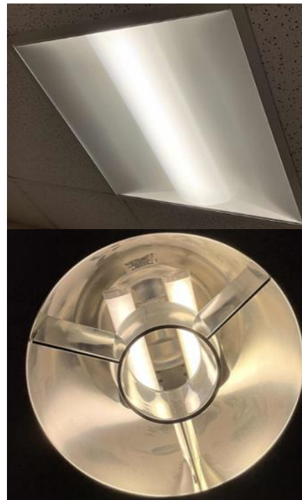
Gym LED High Bay, LED 2x2 & LED Recessed Lamps
