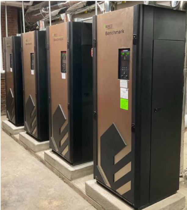
Condensing Boilers
