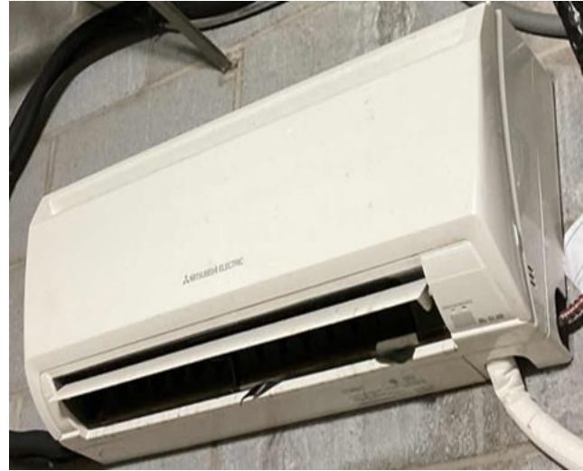
Ductless Split Systems AC
