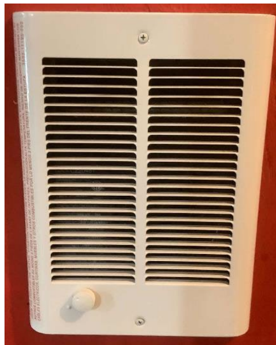
Electric Resistance Heater
