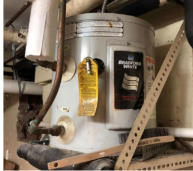
Storage Tank Water Heater
