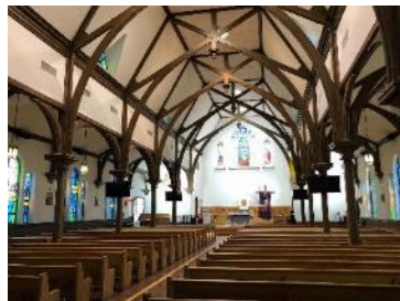
Interior Truss System
