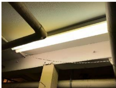
Linear T-12 Light Fixture, Sanctuary
