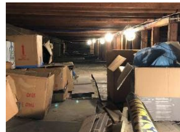
Crawl Space Under Sanctuary
