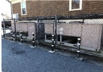
Outdoor Condensing Units
