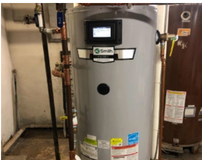
Storage Tank Water Heater
