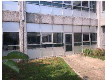
Windows and Exterior Doors
