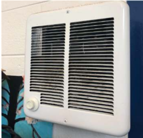
Electric Resistance Heater
