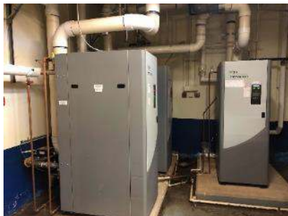
Hot Water Boilers
