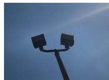
Pole Top Light Fixtures
