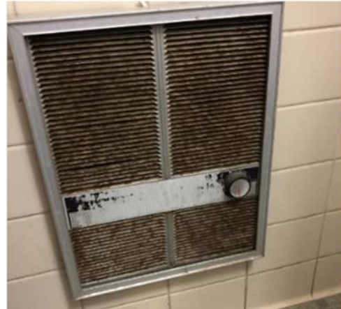
Electric Resistance Heater
