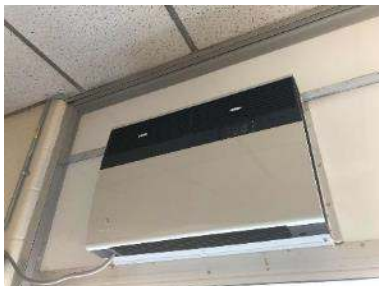
Window AC Unit
