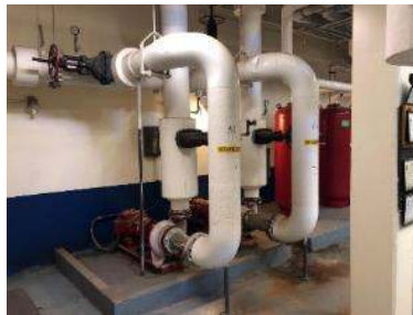
Heating Hot Water Pumps
