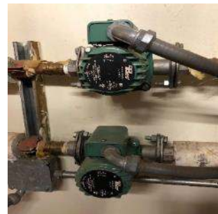
DHW Circulation Pumps
