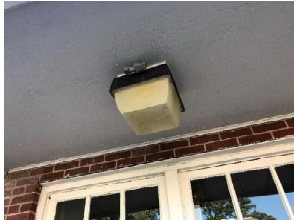
Metal Halide Exterior fixture
