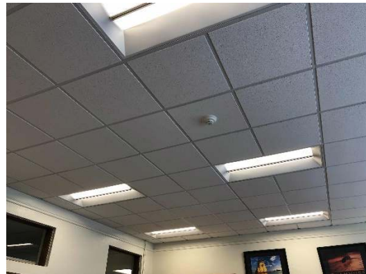
Classroom 4-foot LED Fixtures
