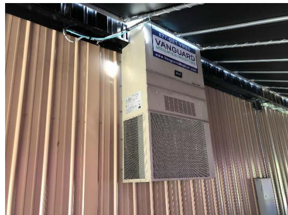
Trailer HVAC Unit
