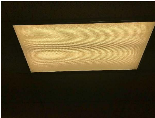
Classroom – 4-foot T8 Troffers
