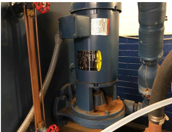
Boiler Feed Water Pump
