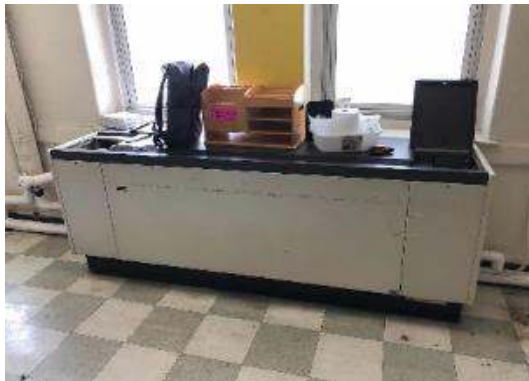
Newer Unit Ventilator
