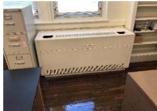
Older Unit Ventilator
