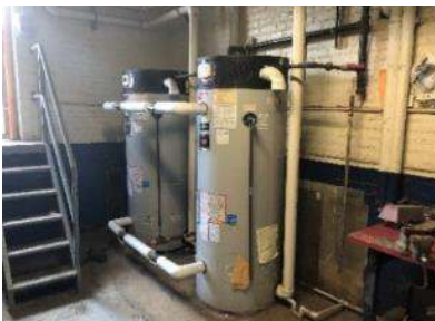
Hot Water Storage Tank
