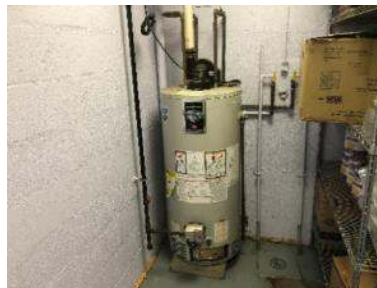
Hot Water Storage Tank
