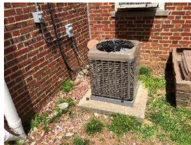
Outdoor Condensing Unit
