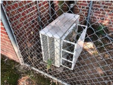
Outdoor Condensing Unit
