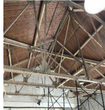
Interior Structural Steel with Wood Decking
