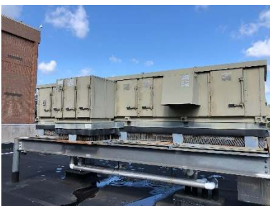
Rooftop Air Handling Unit
