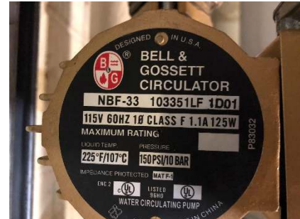
DHW Circulation Pumps
