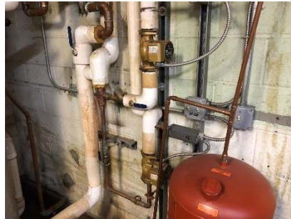
Hot Water Storage Heater
