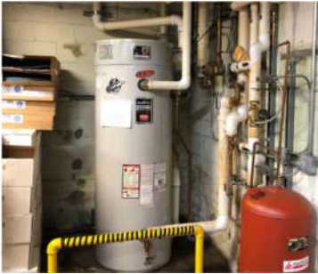
Hot Water Storage Heater
