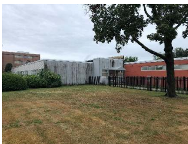
Building Exterior Façade
