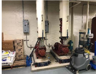
Heating Hot Water Pumps
