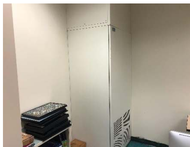
Classroom Air Handling Unit
