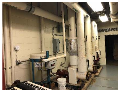
Chilled Water Pumps
