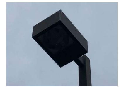
Pole Top Fixture with LED Lamps
