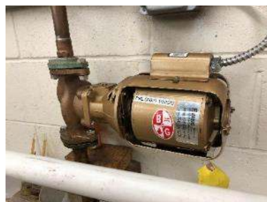
DHW Circulation Pump
