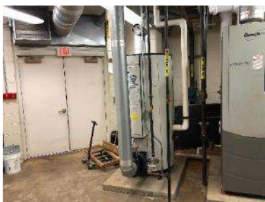
Building Storage Water Heater
