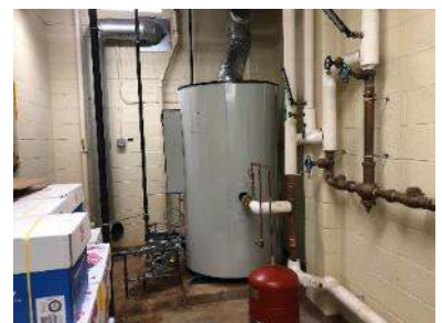
Kitchen Storage Water Heater
