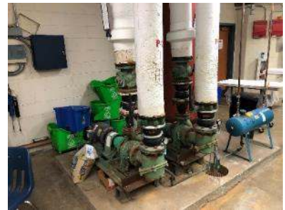
Heating Hot Water Pumps
