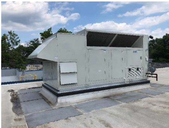
30-ton AAON Unit
