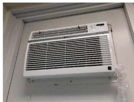
Window AC Unit - Office
