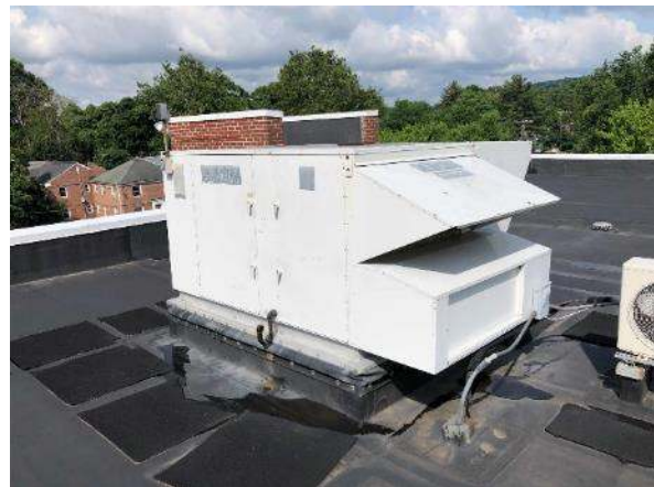
15-ton AAON Unit
