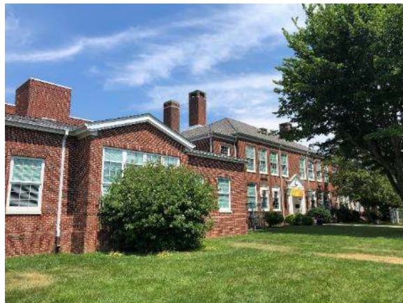
Single and Two-story Facade
