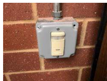
Wall Switch Occupancy Sensor
