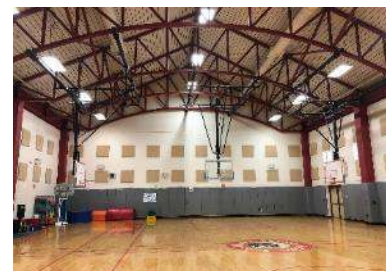
Interior Truss System
