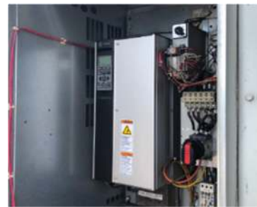
VFD Motor Control
