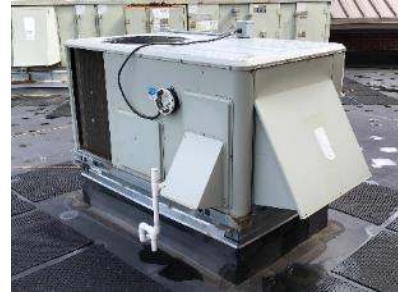
RTU on Roof Near Library
