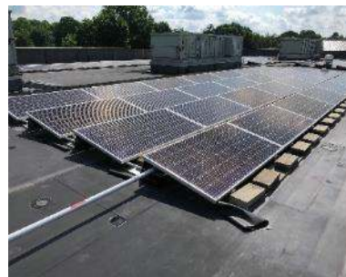
Solar Array on Upper Roof
