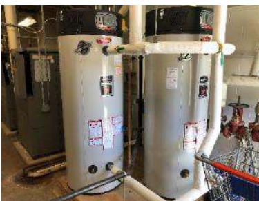
Storage Tank Water Heaters
