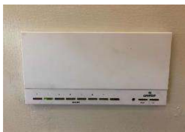
Cafetorium Dimming Controls
