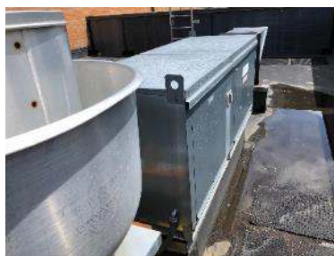
Electric Forced Air Furnace
