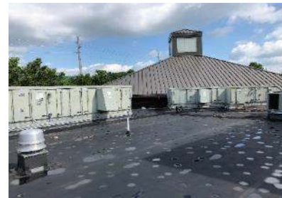
Rooftop Air Handling Units
