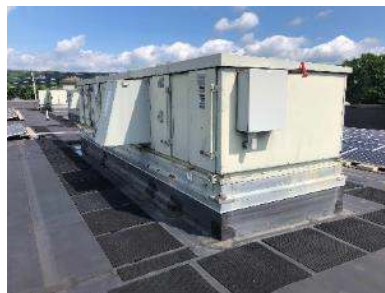
Air Handling Unit
