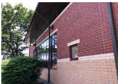
Building Brick Façade
