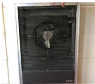
Electric Resistance Heater
