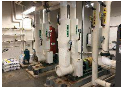
Chilled Water Pumps
