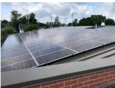
Solar Array on Lower Roof
