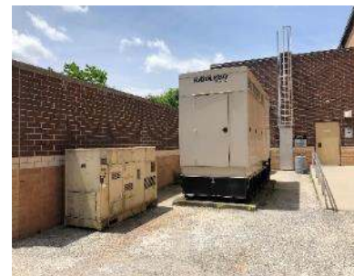
Emergency Back-up Generator
