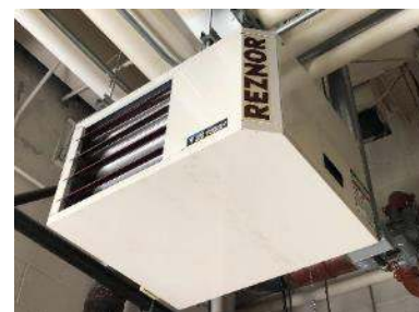
Gas-fired Unit Heater
