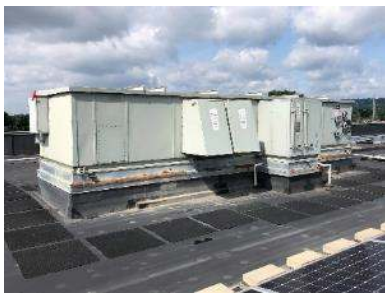
Air Handling Unit
