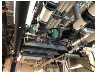
Heating Hot Water Pumps
