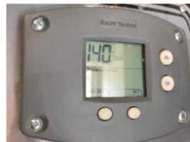
Temperature Setting on Water Heater
