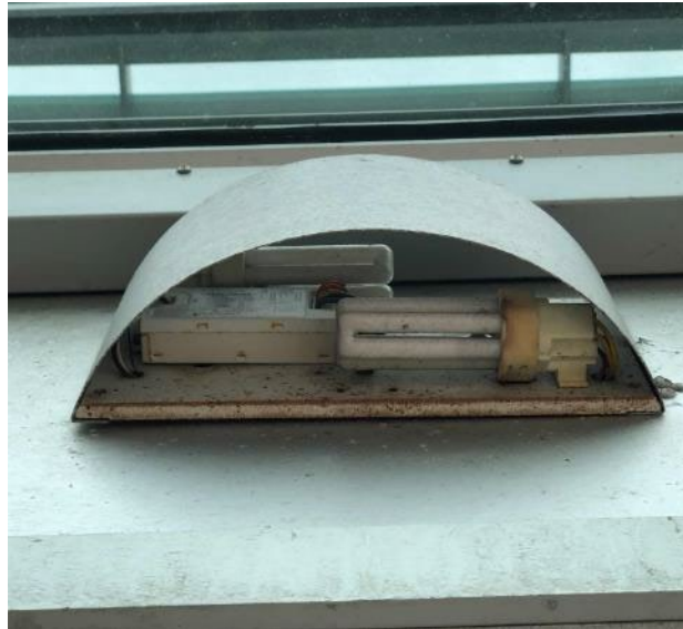
Wall Mounted Fixture with CFLs
