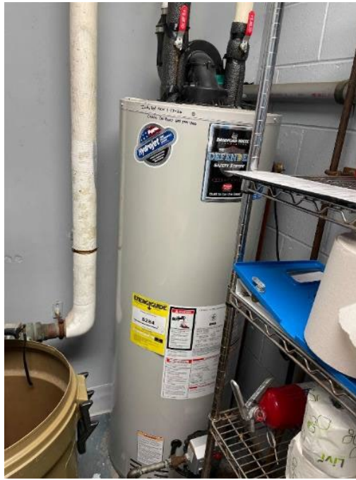
Storage Water Heater
