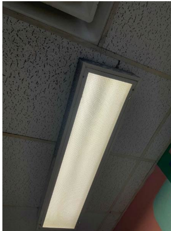
Linear Fluorescent Fixture
