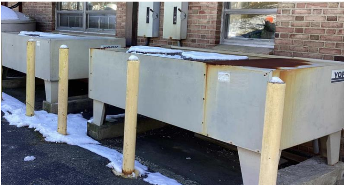
Outside Condensing Units
