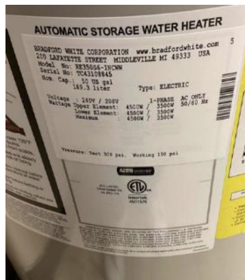
Electric Domestic Hot Water Heater
