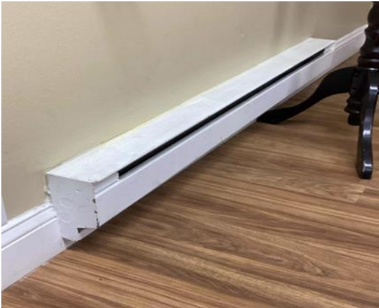
Typical Electric Resistance Heater & Local Thermostat
